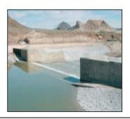
Weirs are low dams designed to reduce streambed erosion by flattening the slope of the channel and slowing flows. Many weirs are constructed of confined rock riprap, providing a somewhat natural look (top). Other structures are built with concrete, resulting in a more engineered look (bottom). Weirs, wetland restoration, and invasive vegetation removal helped reduce total suspended solids (TSS) concentrations in lower Las Vegas Wash and led to its removal from the Nevada 303(d) list in 2004.
