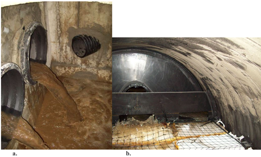
Figure 4: Stormwater entering the treatment device (a.) and moving over the filters (b.)
