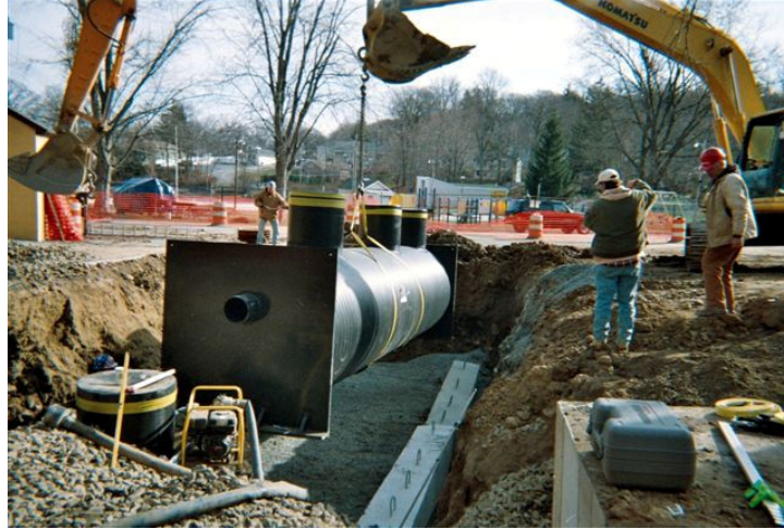
Figure 3: Installation of the Aquafilter Manufactured Treatment Device
