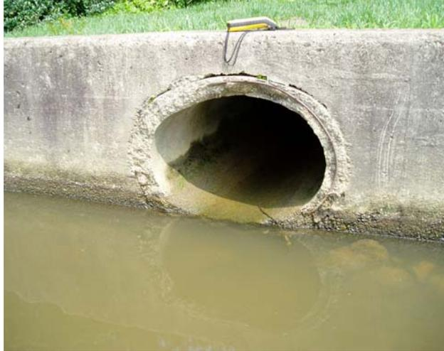
**Figure 9. Storm water outfalls like this one, draining into Brainerd Lake, can contribute to numerous problems such as: elevated nutrient levels, high turbidity, and the exceedance of SWQC for Total Phosphorus.**
