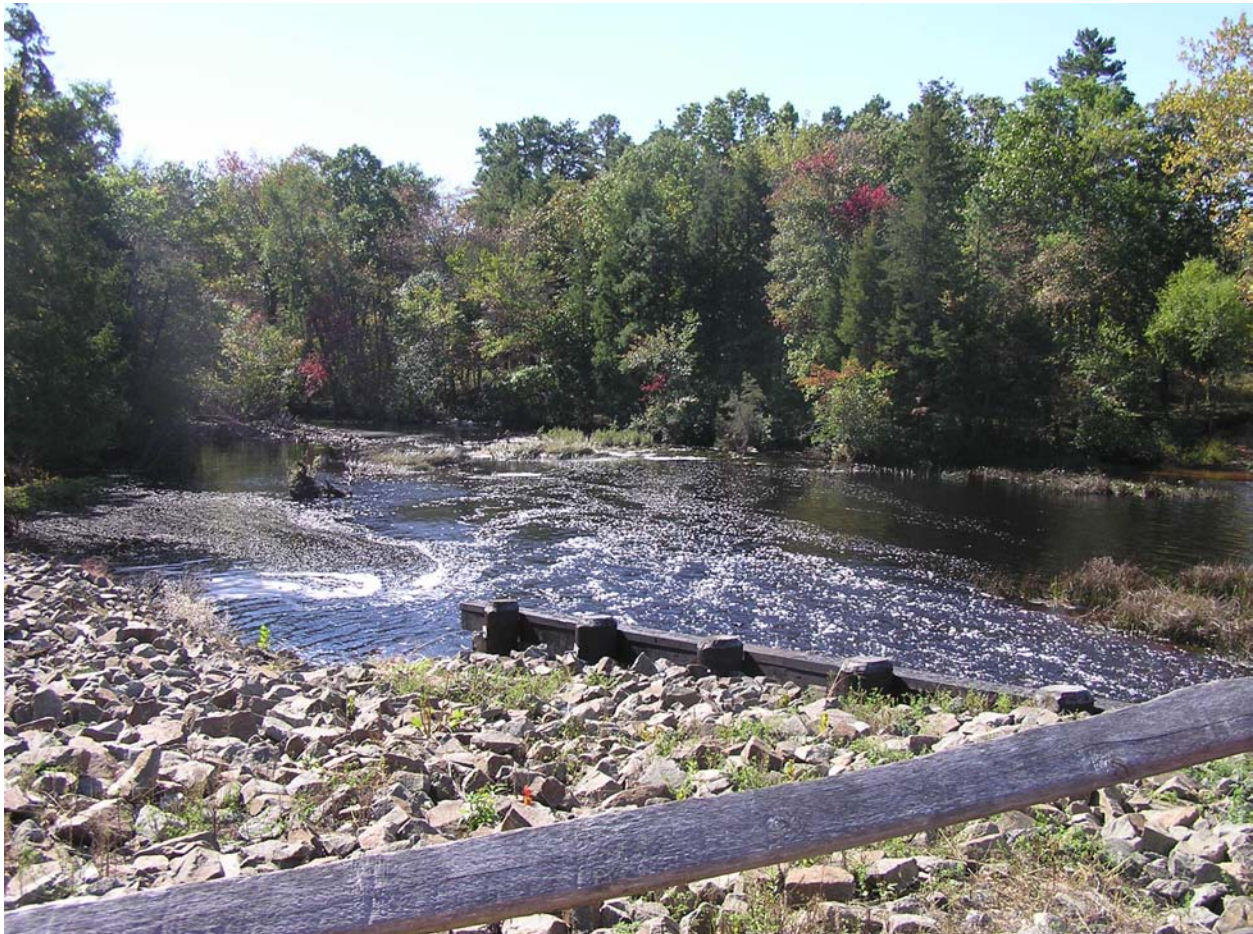
Dam below Batsto Lake, Hammonton, NJ
