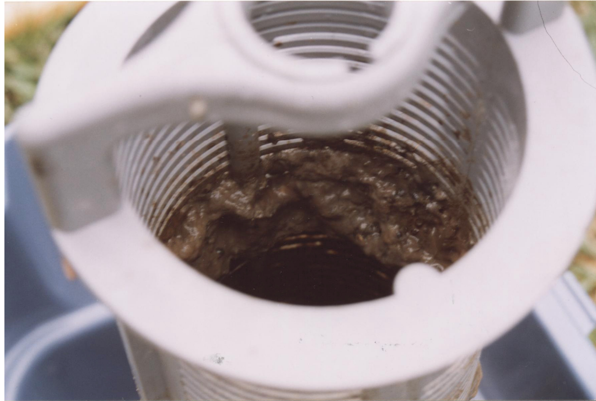
Figure 3. The materials captured in this effluent filter effectively depict what will enter and accrue in the disposal field of an improperly maintained ISSDS (NJDEP).
