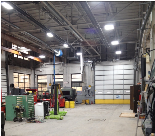
New LED fixtures light up a vehicle maintenance bay at West Orange CSMS.
