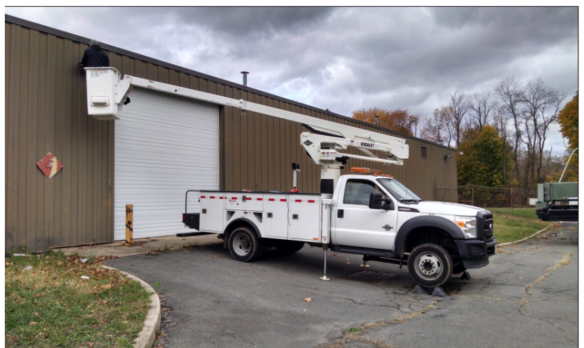
DMAVA electrician, Matthew Scudder, replaces an exterior metal halide light fixture with a new LED. The new LED will use 75% less electricity!
