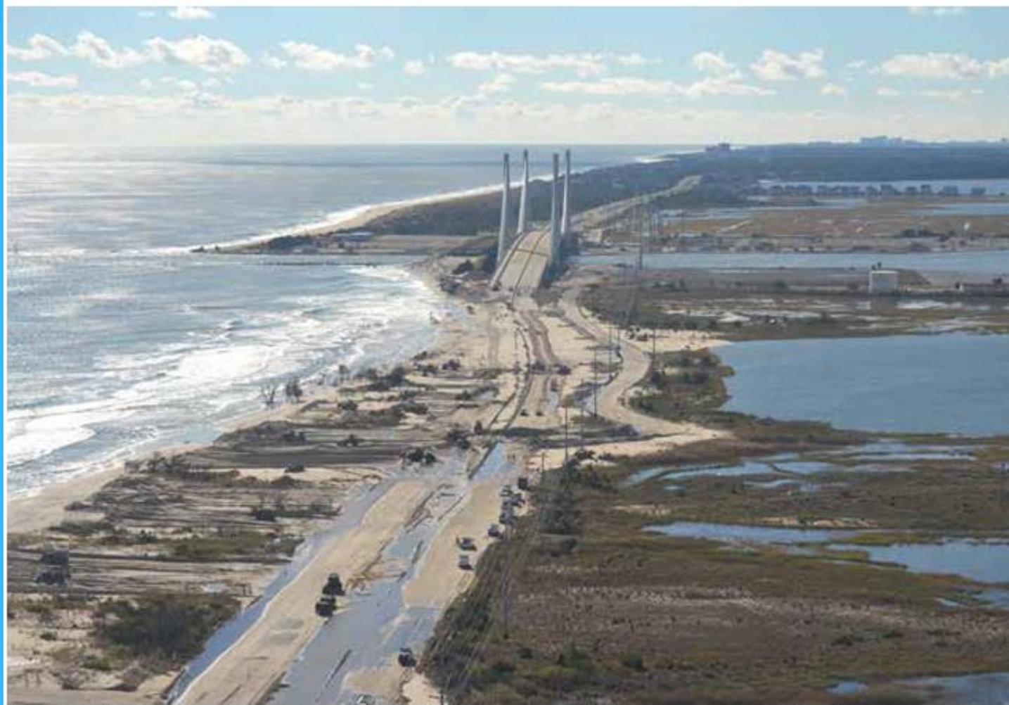
Route 1 at the Indian River Inlet was impassable after Superstorm Sandy due to major dune erosion. Extreme weather events, along with more costly storm damage, are projected to become more frequent as a result of climate change.
