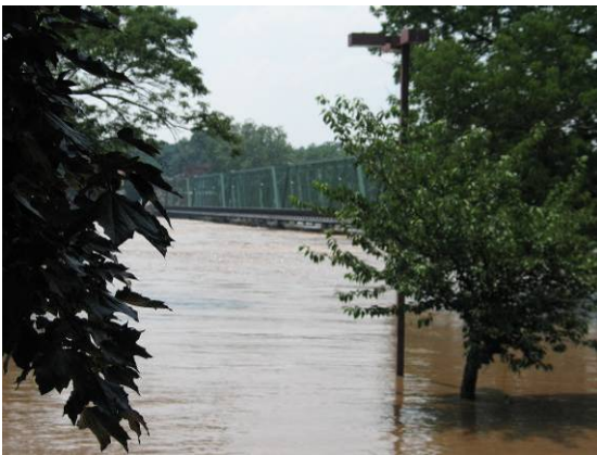
Figure 3.1 Lambertville-New Hope Bridge
