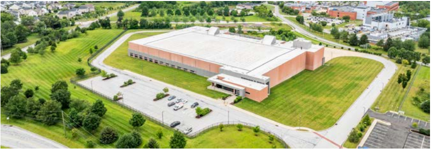
An existing data center located in Collegeville, Montgomery County, PA. Image Source: CoStar Realty Information, Inc.
