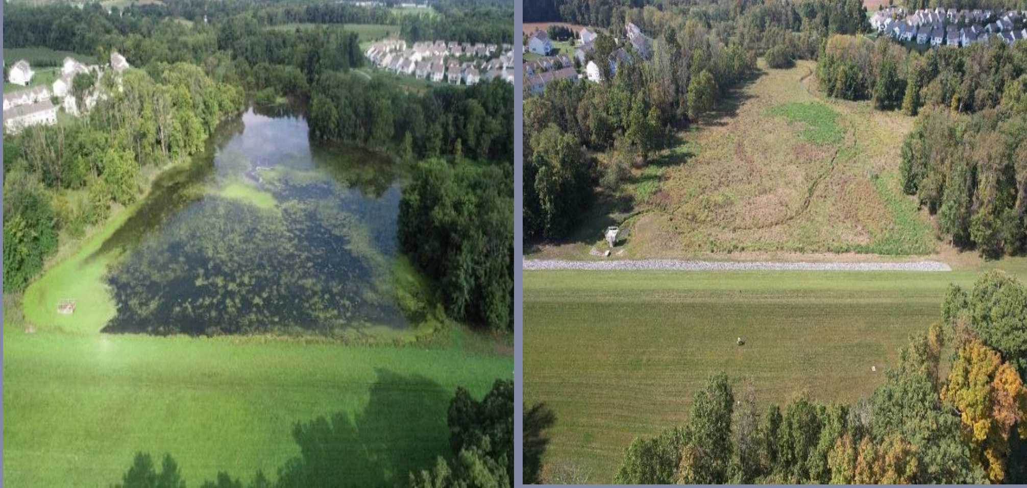
Beaver Creek Dam in East Brandywine Township before (with a 7.2 million gallon pool) and after (operating as dry dam with no permanent pool) the rehabilitation project, completed in 2022.
