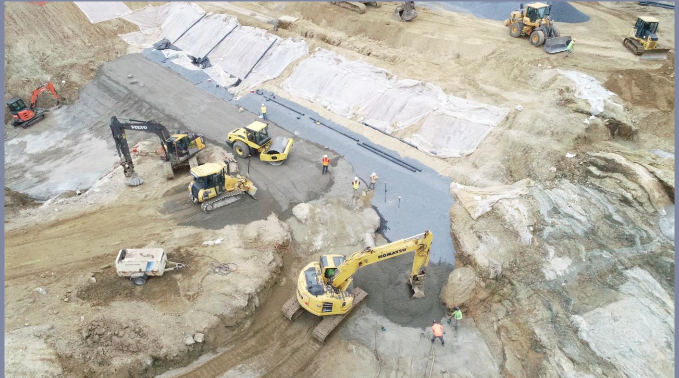
Rehabilitation of Beaver Creek Dam in East Branch Brandywine Creek Watershed, 2021
