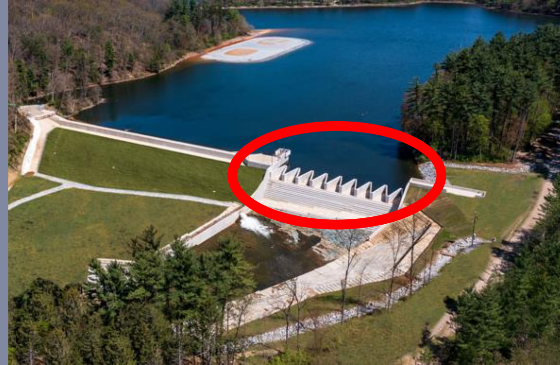
A labyrinth weir constructed at Lake Williams Dam in York, PA (photo courtesy of Gannett Fleming)
