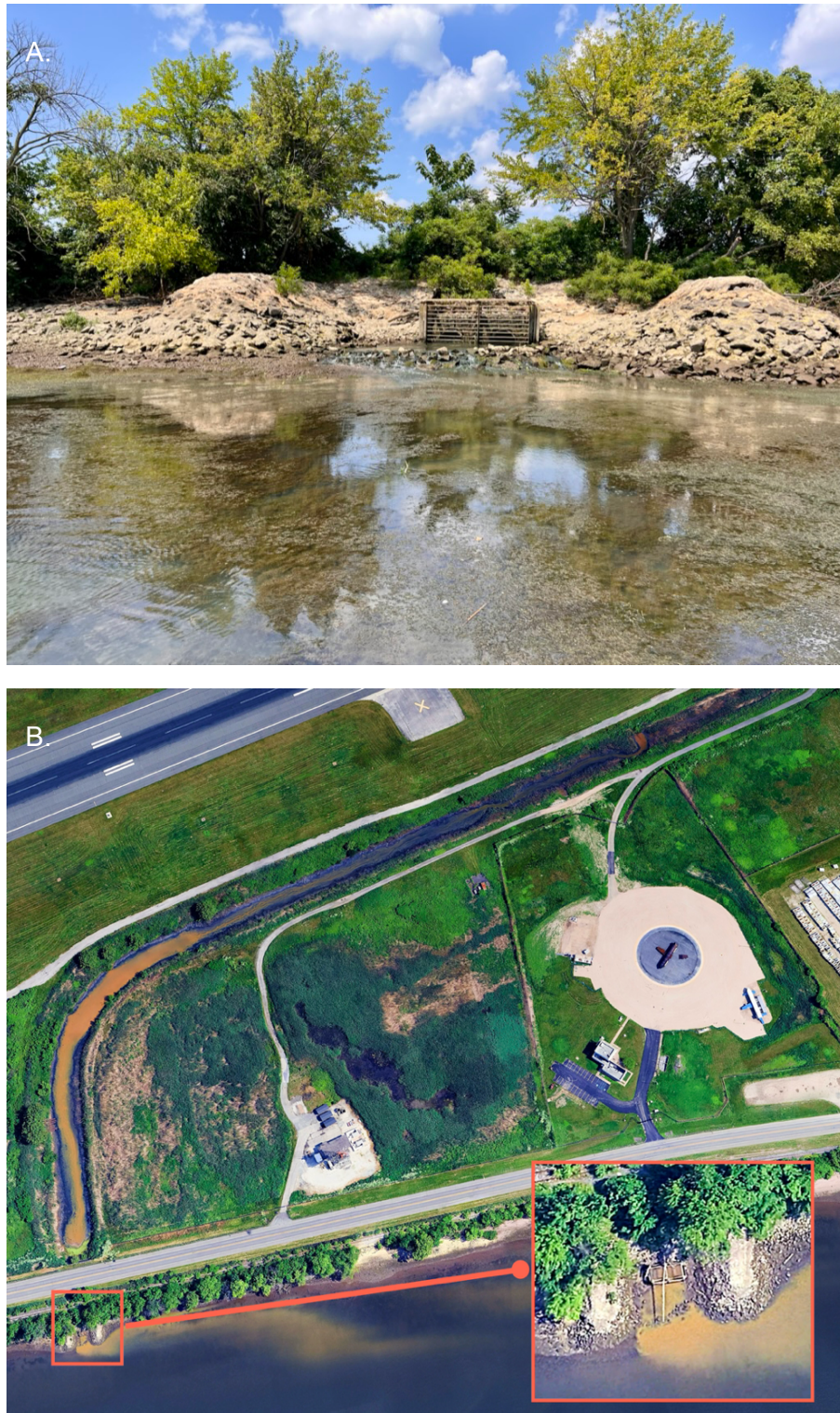
Figure 9. A) The stormwater outfall where the Philadelphia Airport sample was collected. B) View of the stormwater outfall from a Google Earth image that shows the proximity to the firefighting training facility.
