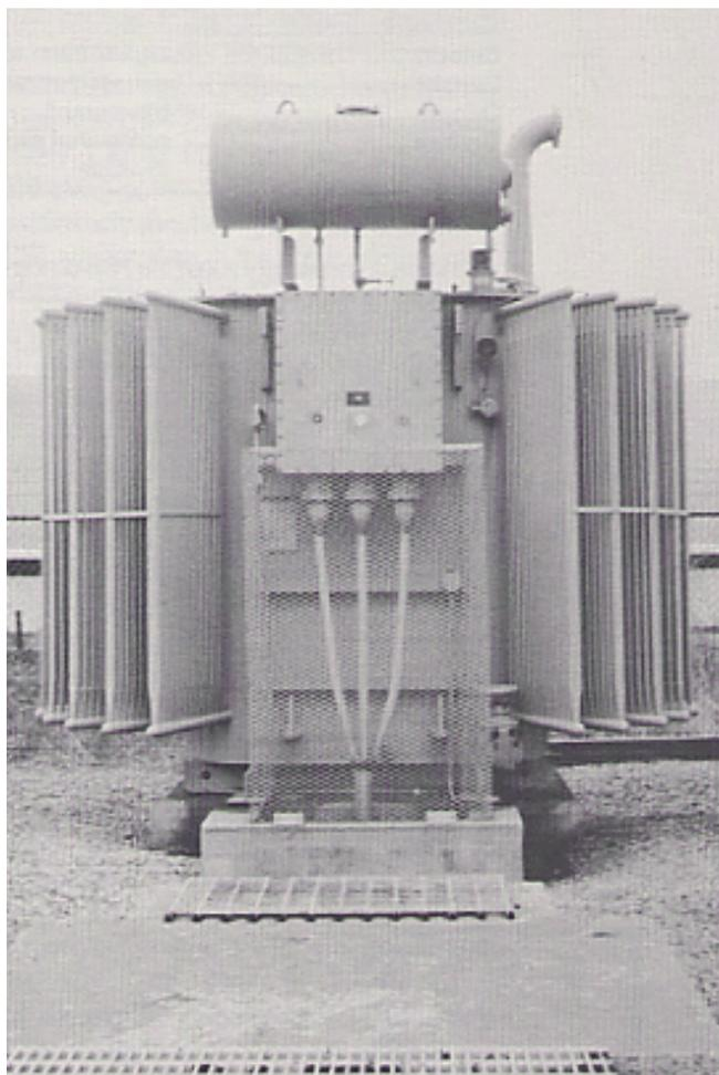
**Figure 3 Liquid-filled Transformer with Conservator Tank**
