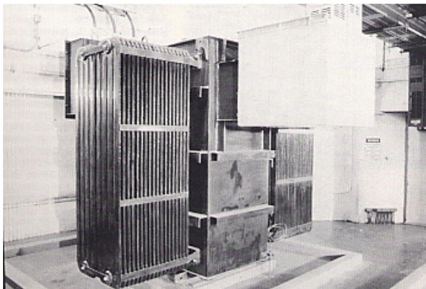
**Figure 1 Liquid-filled Transformer
