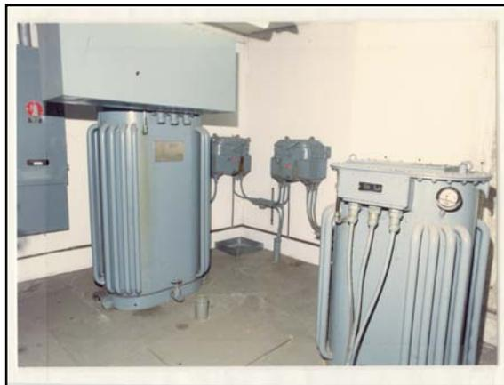
Figure 4-1. Two PCB Transformers.
