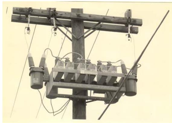
Figure 4-3. Six large high voltage capacitors.
