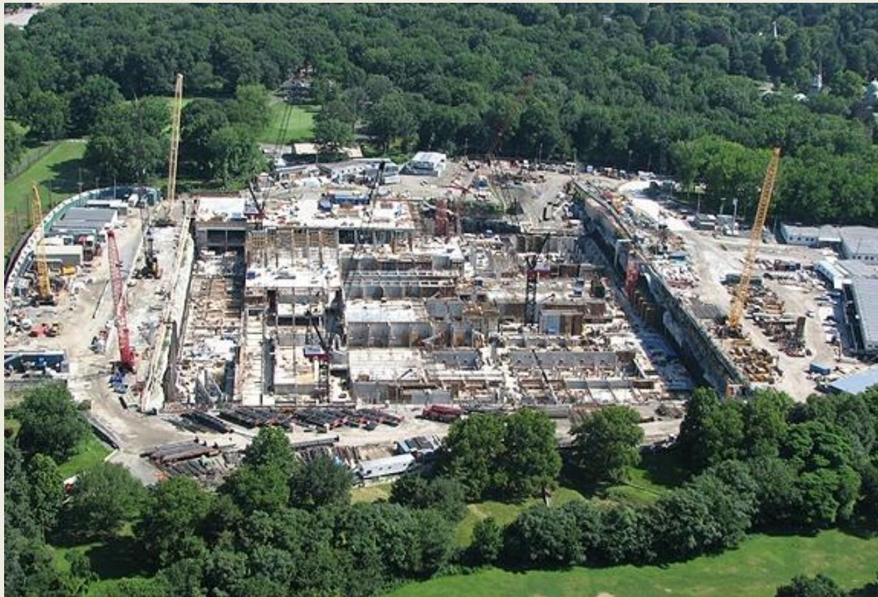
The **290** mgd capacity of the Croton Water Treatment Plant will provide high quality water from the Croton system, and will restore the **240** mgd of lost Croton system safe-yield to the NYC water supply system.
