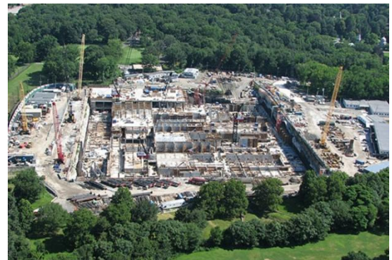
The Croton Water Treatment Facility under construction
