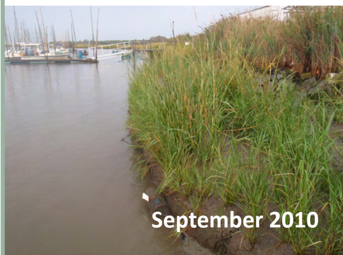
Fig. 5.32. Installation of a mussel and plant-based living shoreline to help stabilize erosion and improve ecological value of a formerly hardened shoreline at Matt's Landing, New Jersey. This new tactic was developed jointly by the Rutgers Haskin Shellfish Research Laboratory and Partnership for the Delaware Estuary. The photo from Sept 2011 was following Hurricane Irene and Tropical Storm Lee
