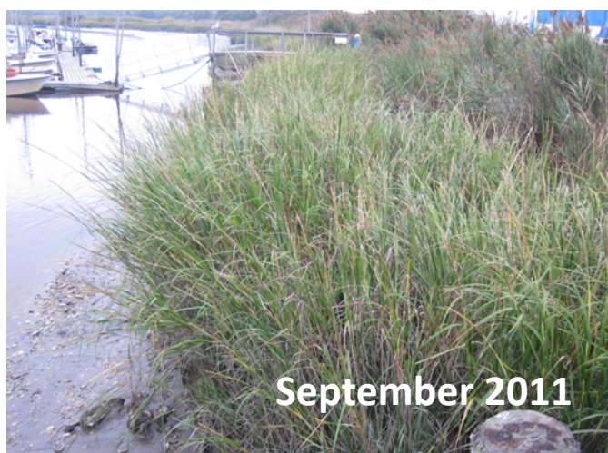
Fig. 5.32. Installation of a mussel and plant-based living shoreline to help stabilize erosion and improve ecological value of a formerly hardened shoreline at Matt's Landing, New Jersey. This new tactic was developed jointly by the Rutgers Haskin Shellfish Research Laboratory and Partnership for the Delaware Estuary. The photo from Sept 2011 was following Hurricane Irene and Tropical Storm Lee
