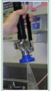
**NEW: Pre-Rinse Spray Valves** (≤ 1.28 gpm)
