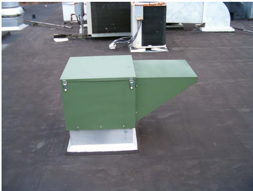
Photograph 2: Positive pressure fresh air intake located on roof top of shopping center business.
