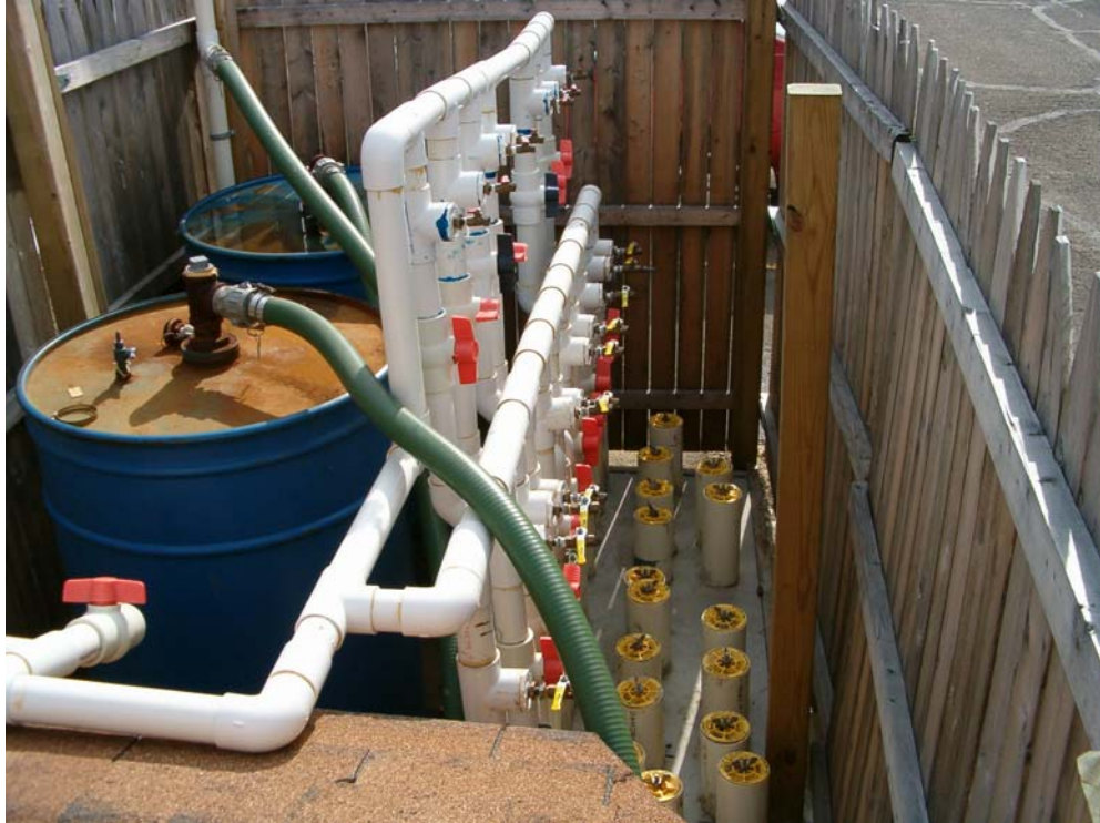
Photograph 3: Soil venting system located at the south end of the shopping center.
