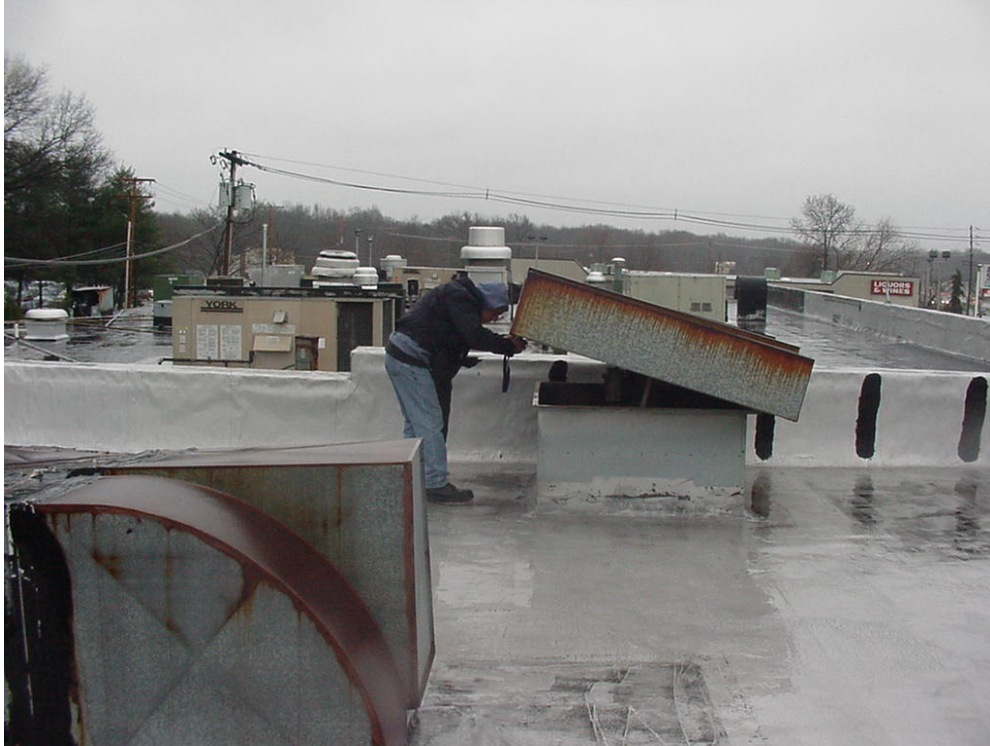
Photograph 6: Roof top exhaust vent for Tops 'N' Town Cleaners.
