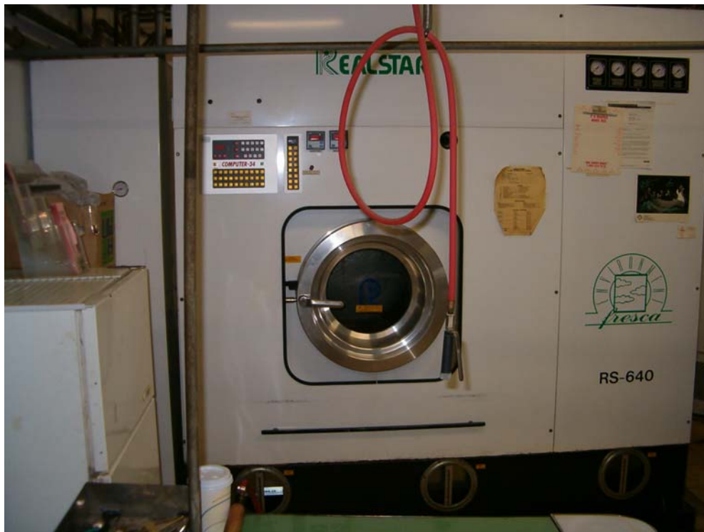
Photograph 4: Realstar RS-640 dry cleaning machine within Tops 'N' Town Cleaners.
