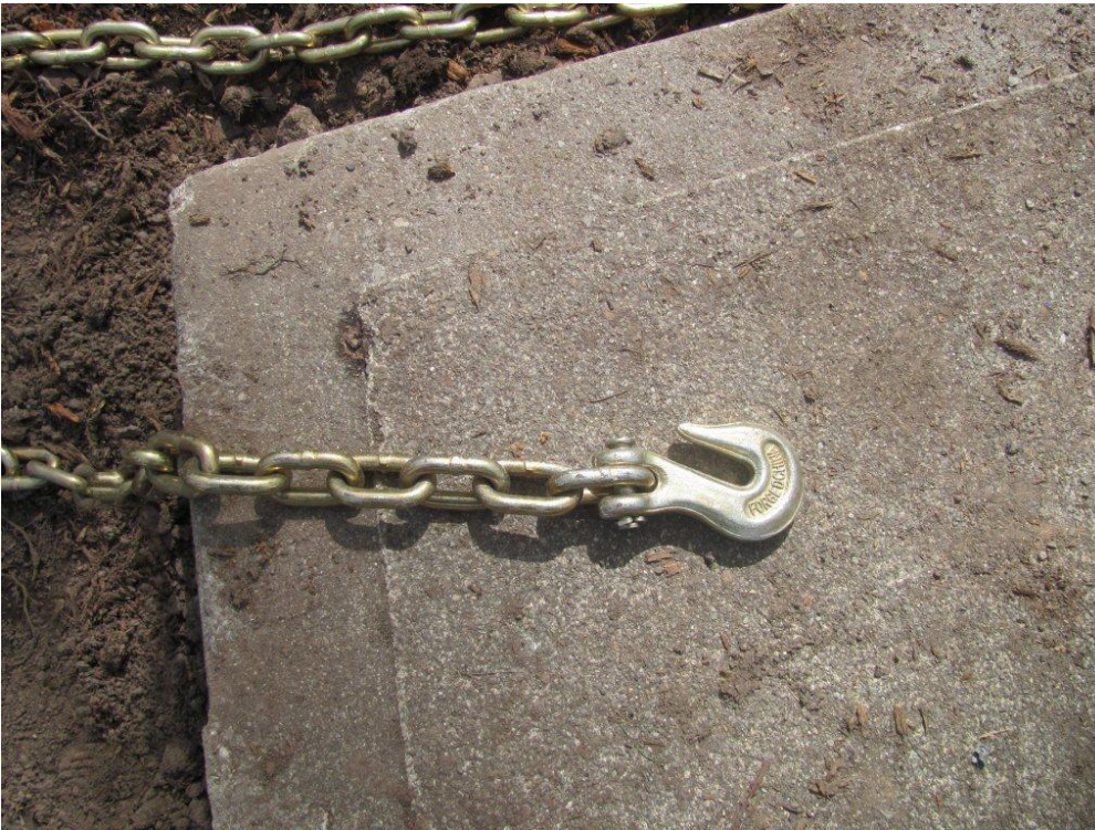
FIGURE 3. Chain with two-inch pelican hook used to lift the slab.
