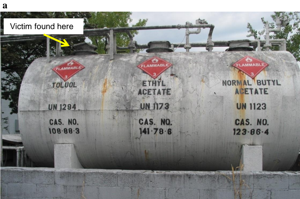
FIGURE 1: Incident site, above-ground storage tank with three 2,000-gallon sections (a. side view; b. front view).
