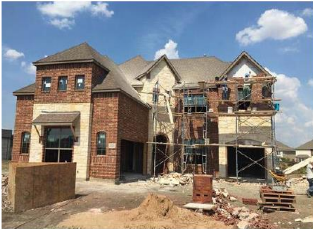
Crews construct a Ryland Group home near Dallas.
