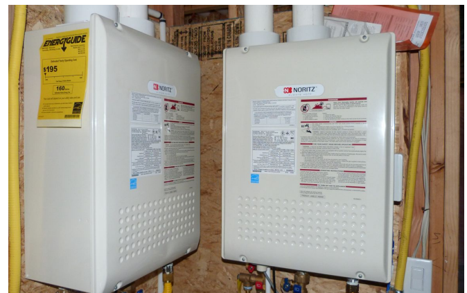
Figure 3. Tankless Water Heater
