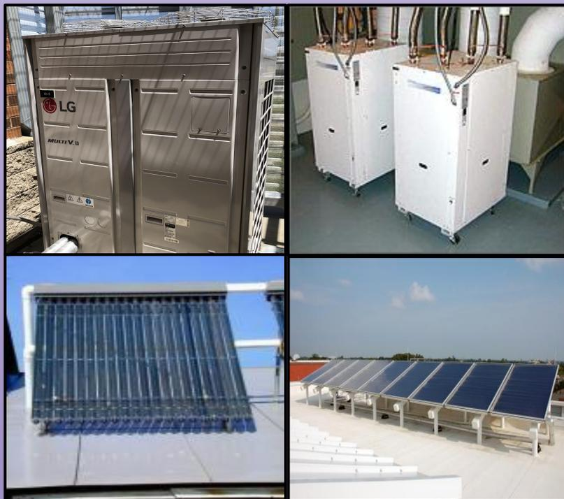
*Clockwise from top left: Air source heat pump, ground source heat pump, evacuated tube solar collector for hot water heating, and flat plate solar collector for hot water heating*
