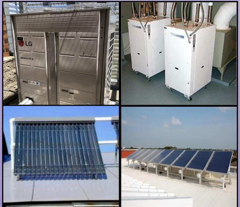
*Clockwise from top left: Air source heat pump, ground source heat pump, evacuated tube solar collector for hot water heating, and flat plate solar collector for hot water heating*
