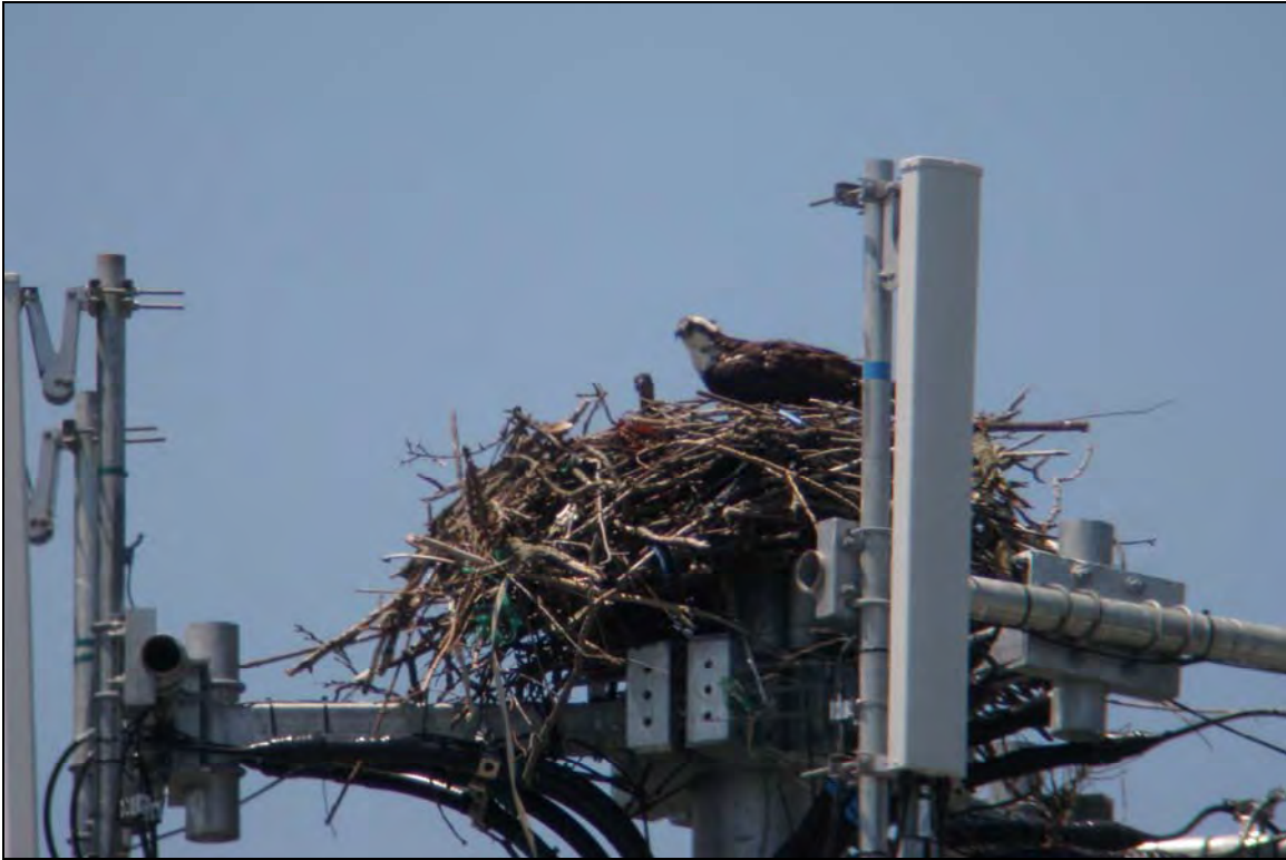
Photo C: View of osprey nest on cell tower. At 1:00 pm one adult osprey and one chick were observed in the nest on the cell tower.
