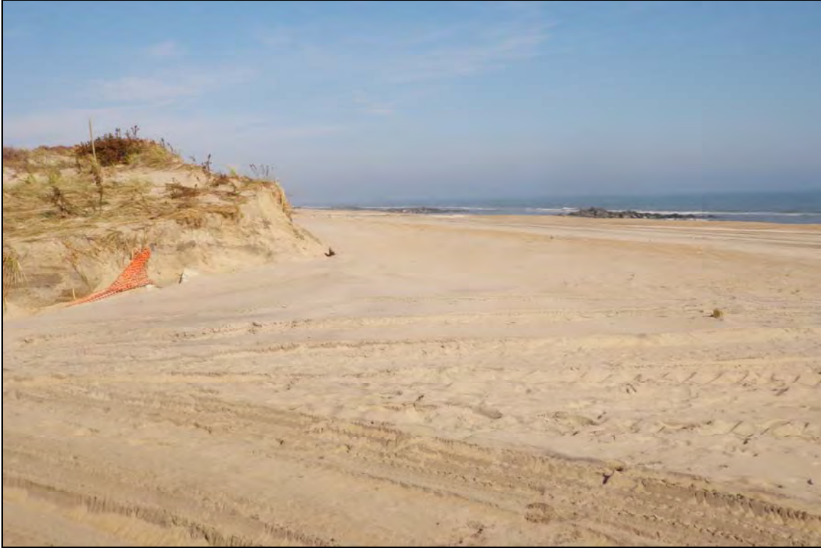
Photo C: View northeast of the corner of the Southern Beach Area. Note the significant amount of erosion as a result of Hurricane Sandy.
