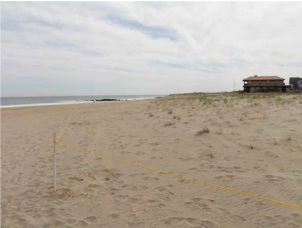
Photo D View of SPA looking south. The frontal portions of the SPA have also lost American beach grass from recent storms.
