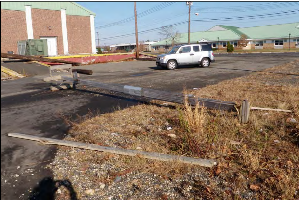
Photo B: View of osprey platform that was installed by ASGECI shown snapped at the base as a result of Hurricane Sandy on October 29, 2012.
