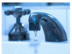
should be reported to the building manager and repaired as soon as possible. These fixtures can be repaired by replacing gaskets, washers, and other components that may deteriorate as a result of frequent use.
