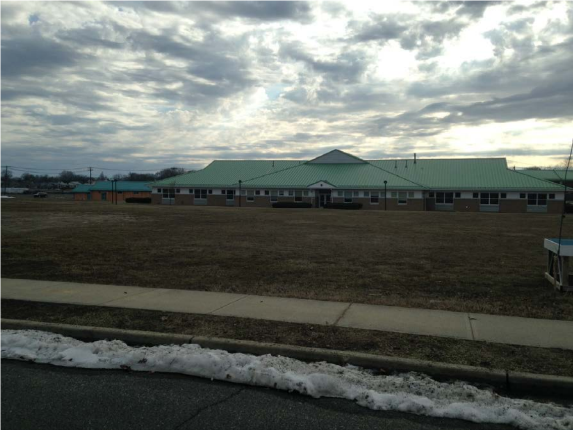
Photograph 4: Location of proposed General Instruction Building/Medical Clinic (GIB/MED), facing south.
