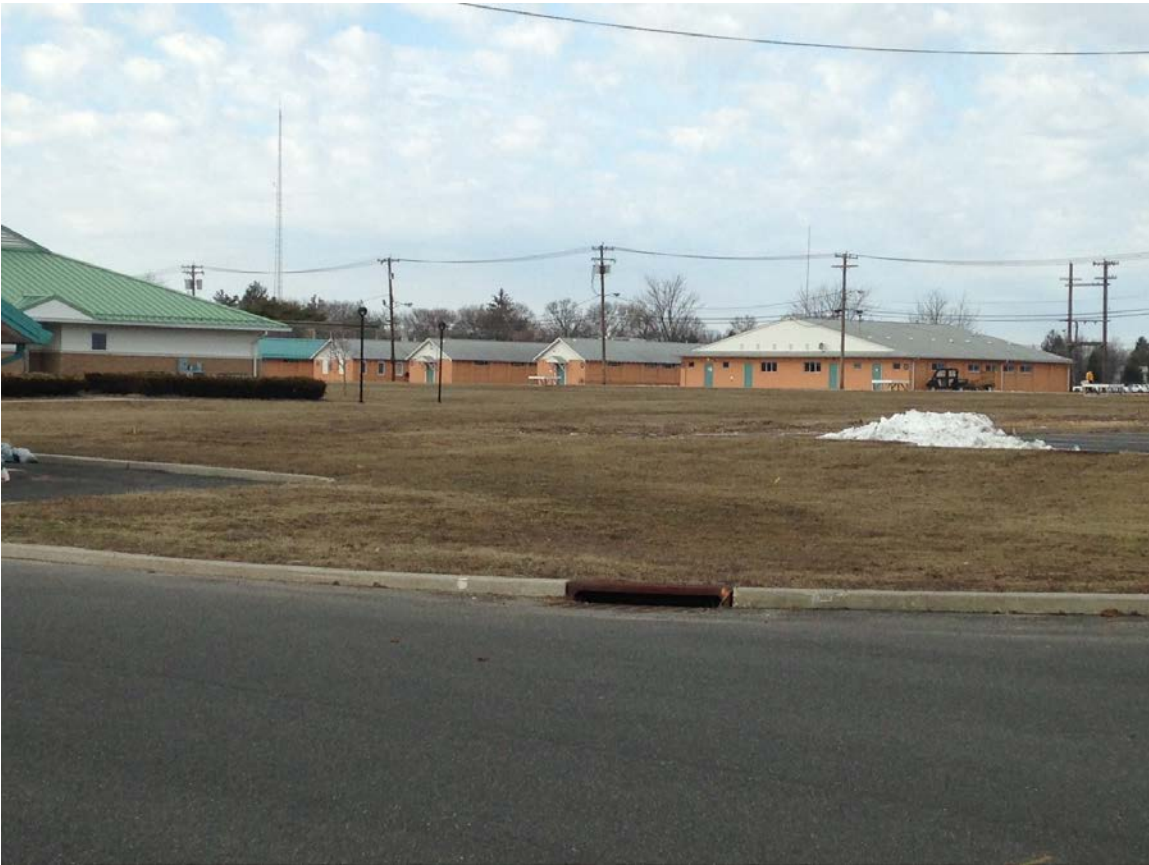
Photograph 3: Location of proposed General Instruction Building/Medical Clinic (GIB/MED), facing north.
