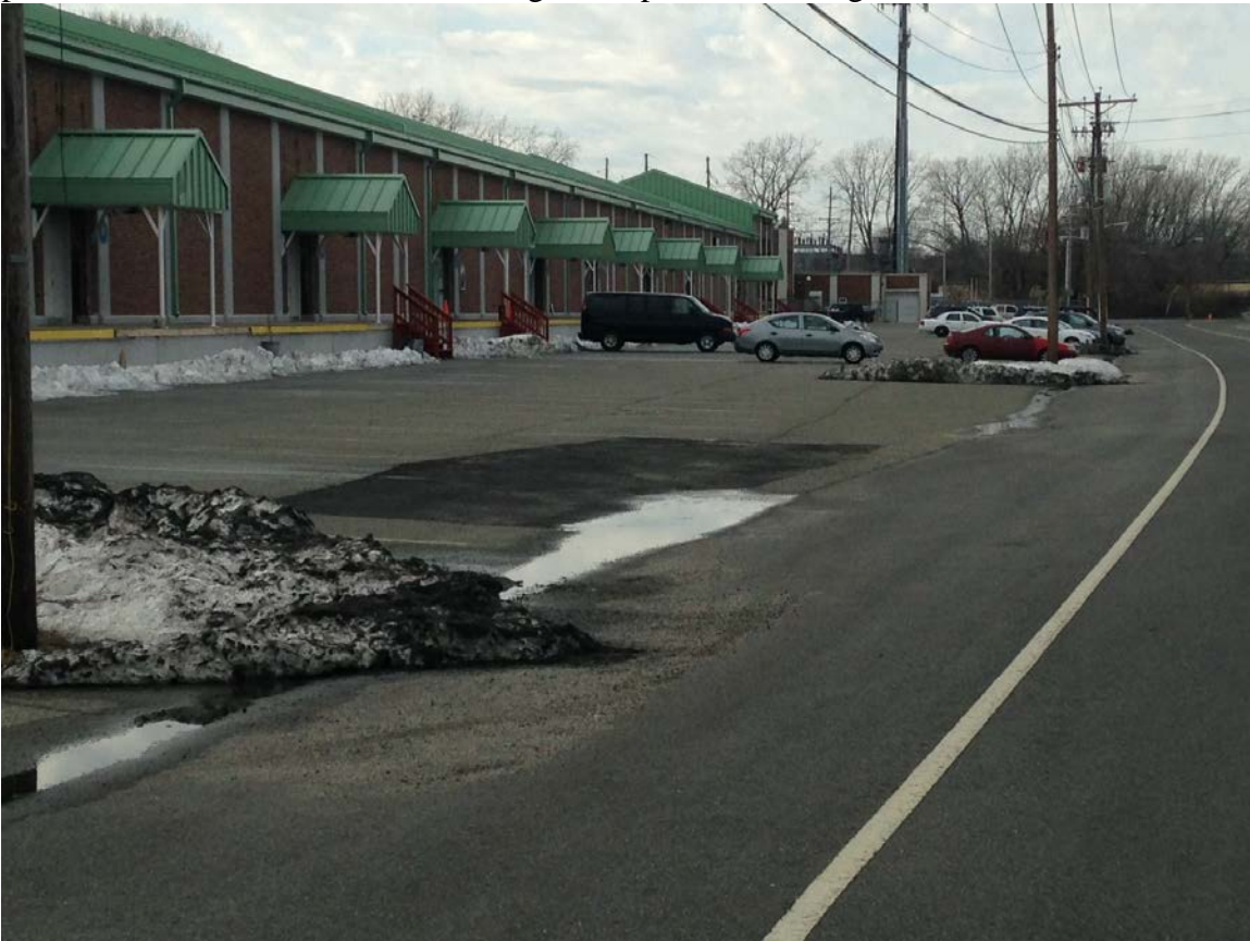
Photograph 8: View of the southwestern portion of the subject property, along Governor Wilson Drive, facing west.
