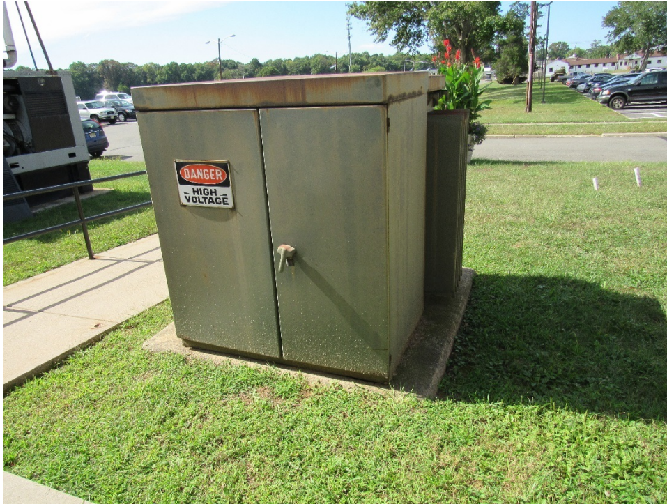
Photograph 12 – An unmarked pad-mount transformer located outside the USPFO/HSCOE building (Figure 13, Map ID 010). Manufacture data is unknown.
