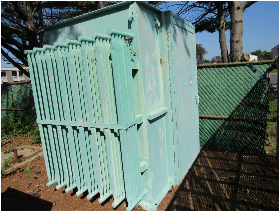
Photograph 23 – An unmarked transformer located outside Building 8. Build is consistent to transformers built in the 1970's and manufacture data is unknown (Figure 16, Map ID 028).
