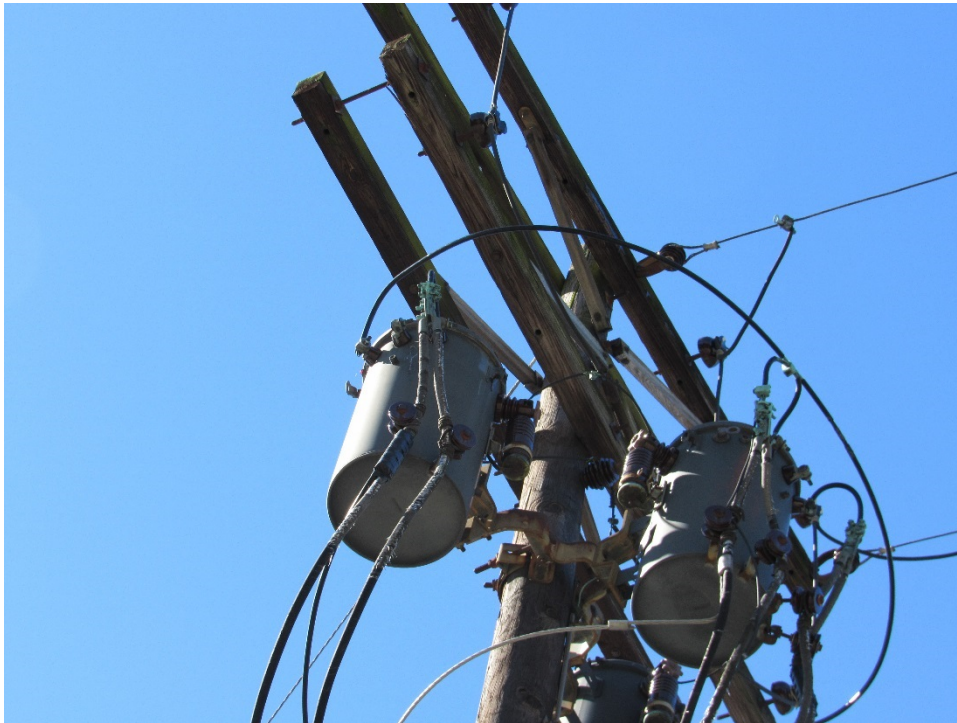
Photograph 30 – Utility pole containing the suspected GE transformer at the Dover facility (also contains two GE transformers manufactured at a non-PCB GE facility) (Figure 23, Map ID 002).
