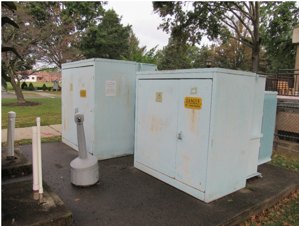
Photograph 9 – Located behind the NJARNG HQ building, the pad-mount transformer in the foreground is believed to be a GE and is suspected to contain PCBs (Figure 13, Map ID 003). The larger transformer in the background is a GE that was sampled in 1986 and confirmed to contain PCBs at 630 ppm (Figure 13, Map ID 002).
