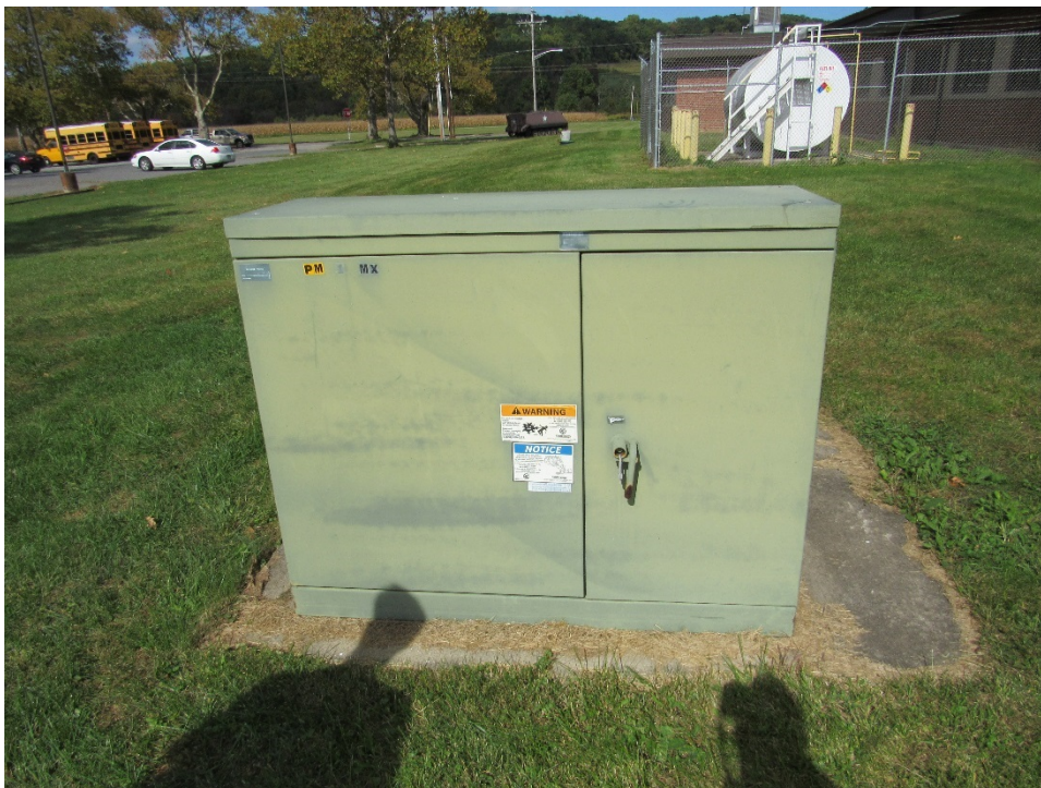
Photograph 36 – The pad-mount transformer (Figure 35, Map ID 001). PCB status could not be determined due to lack of manufacturer data. This transformer is owned by JCP&L.
