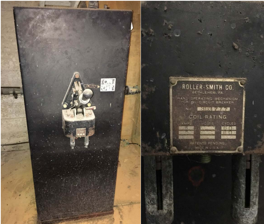
Photograph 1 – The Roller Smith oil switch and associated name plate located in the transformer vault at the Vineland facility (Figure 6, Map ID 002).
