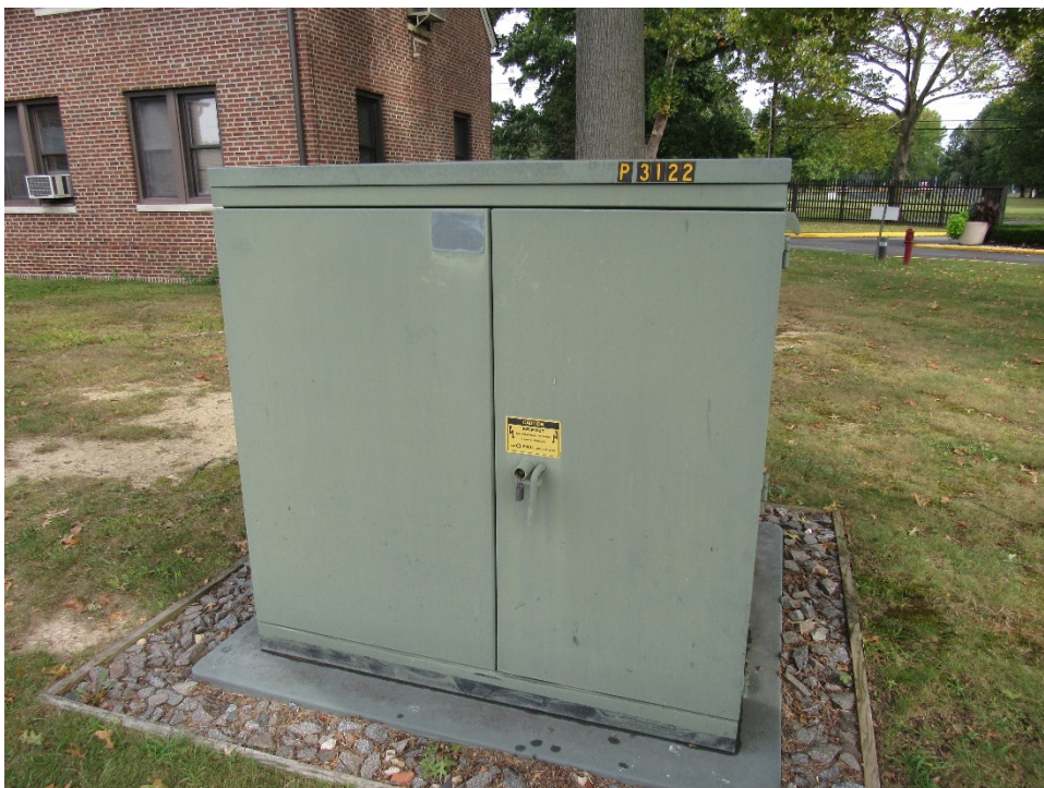
Photograph 11 – A pad-mount transformer located north of the Armory (Figure 13, Map ID 004). PSE&G could not find this transformer in their database. The transformer appears to be a mid-80's build, however, manufacture data is unknown.
