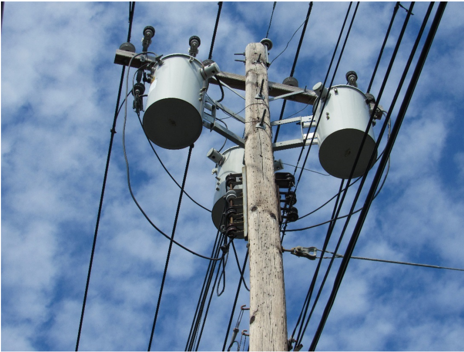
Photograph 21 – The utility pole containing three Westinghouse transformers manufactured in 1976 (Figure 16, Map ID 022).
