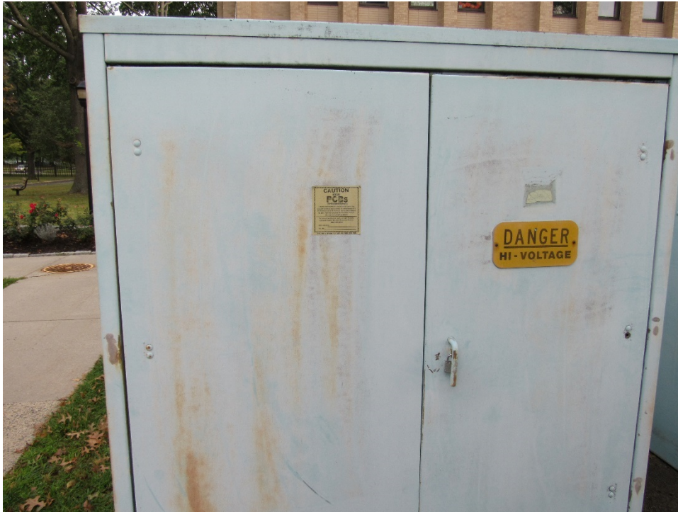
Photograph 10 – Another photo of the GE transformer confirmed to contain PCBs in 1986 (Figure 13, Map ID 002).
