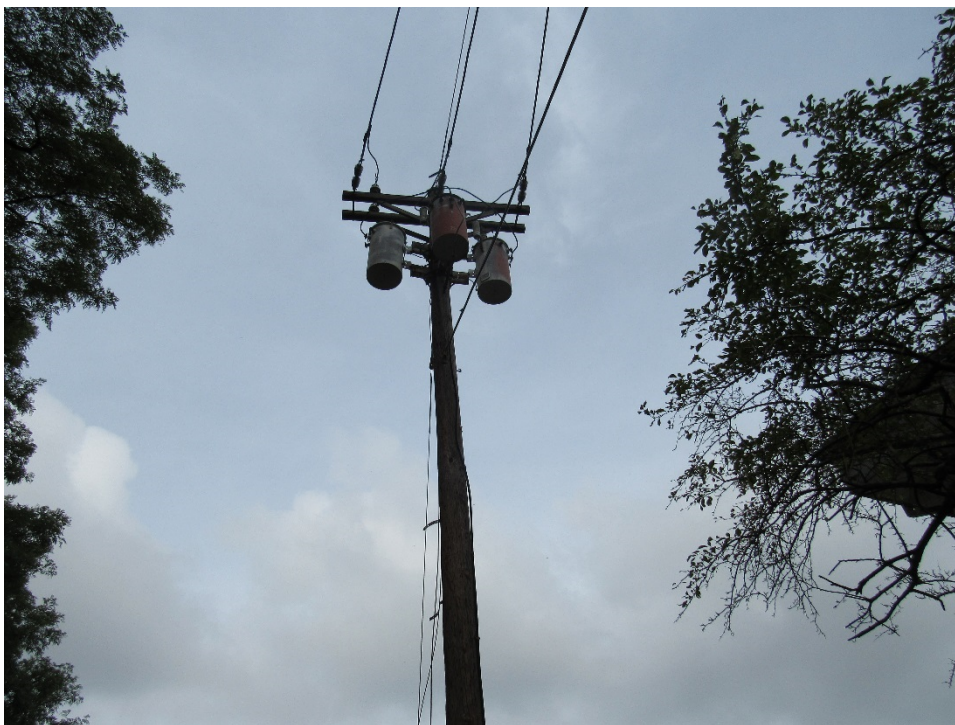
Photograph 2 – Three pole-mount Kuhlman transformers located at the Bordentown Facility (Figure 9, Map ID 002).
