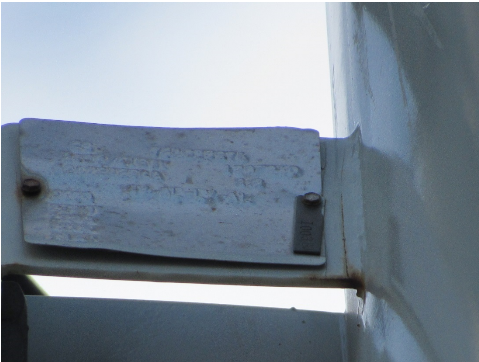
Photograph 22 – The manufacture name plate for the Westinghouse transformer above, the third character of the serial number (which indicates place of manufacture) is illegible (Figure 16, Map ID 022).
