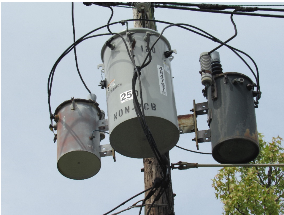
Photograph 13 – The utility pole containing the suspected PCB containing Kuhlman transformer (Figure 13, Map ID 007).
