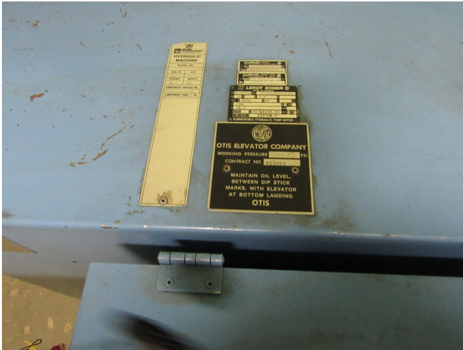
Photograph 35 – The manufacturer name plate for the Otis Elevator Company (Figure 35, Map ID 004). Due to its age the elevator motor is suspected to contain PCBs.
