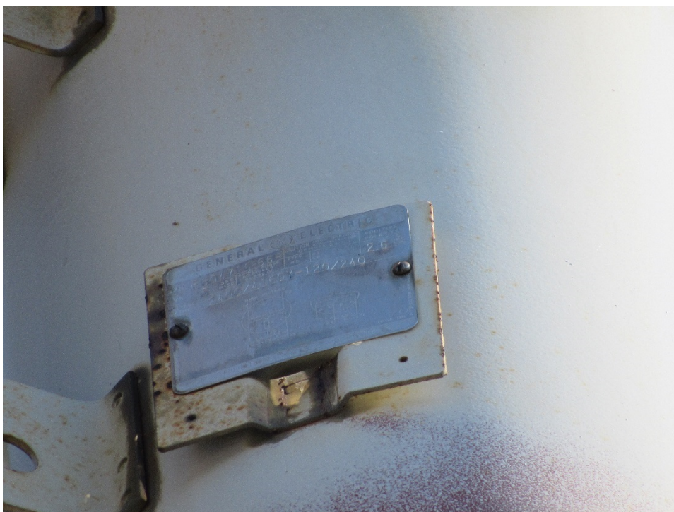
Photograph 20 – The manufacturer name plate on the GE transformer suspected to contain PCBs (Figure 16, Map ID 016).
