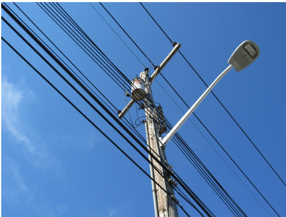
Photograph 19 – The utility pole containing one GE transformer that was manufactured in a GE facility known to have used PCBs (Figure 16, Map ID 016).
