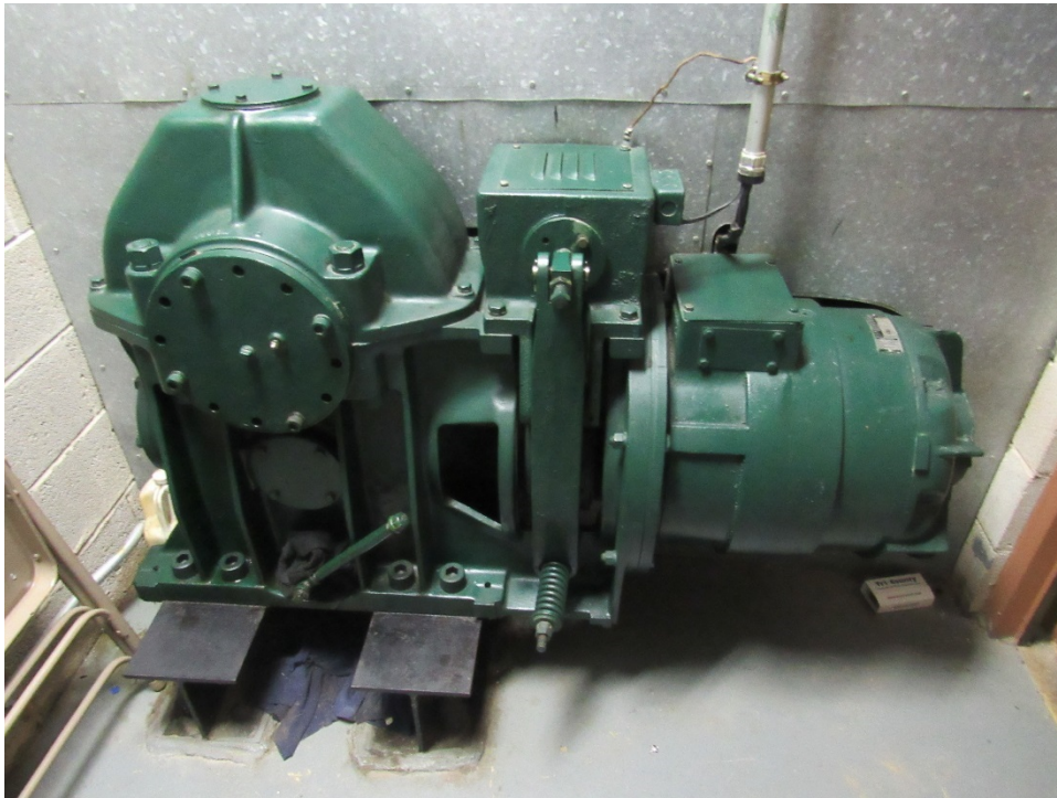
Photograph 8 – The Otis elevator motor located in the basement of the NJARNG HQ building at the Lawrenceville facility (Figure 13, Map ID 001).
