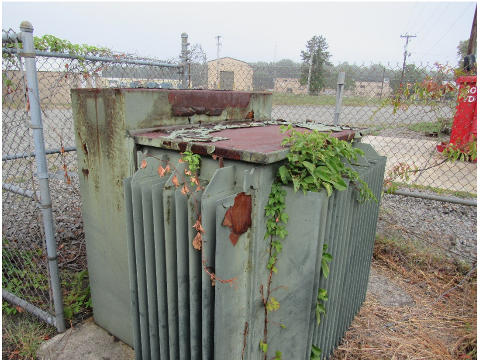
Photograph 7 – Another angle of the pad mount transformer located behind Building 3601 in the secured vehicle yard (Figure 11, Map ID 003).
