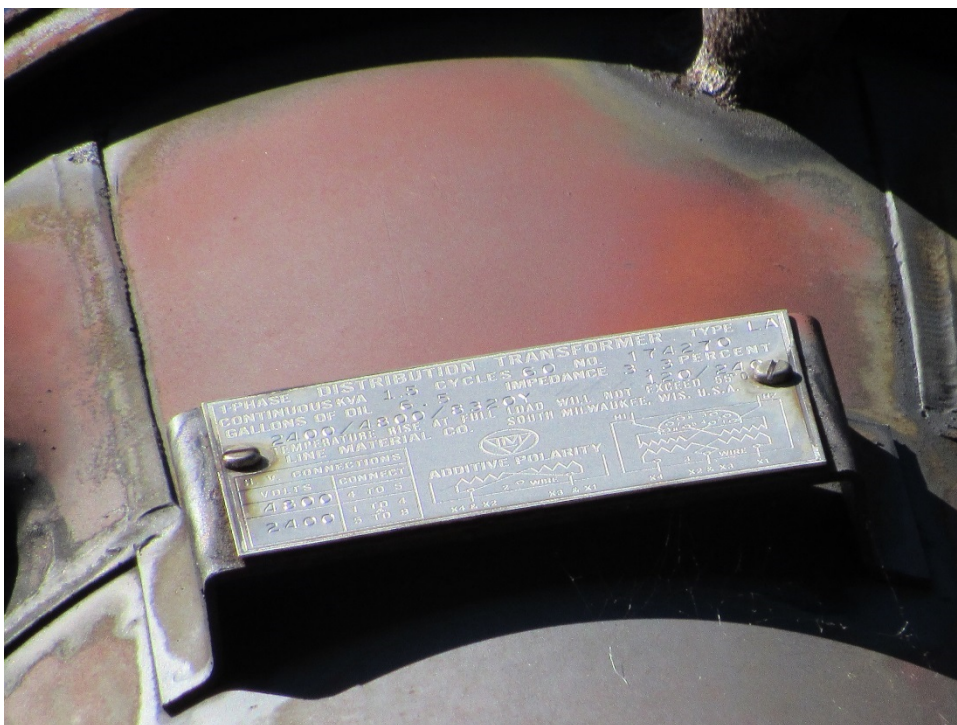
Photograph 29 – The name plate on the Line Material Co. transformer at the Dover facility (Figure 23, Map ID 001).
