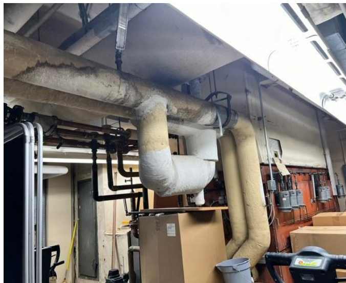
Existing Duct Work
