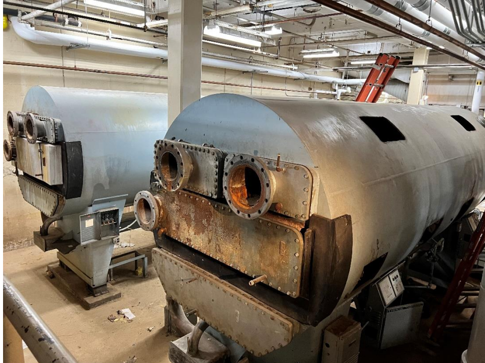
Existing Decommissioned Chillers to be Demolish
