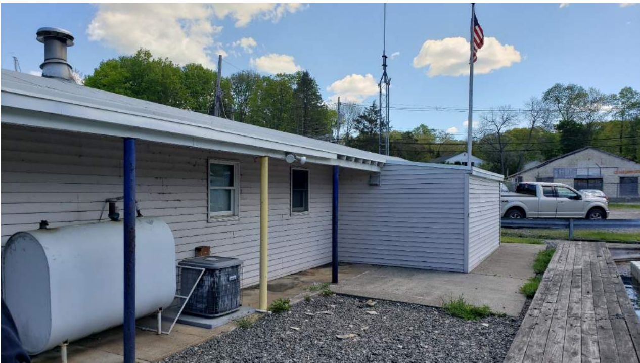
Existing Police Station Building – South Façade
