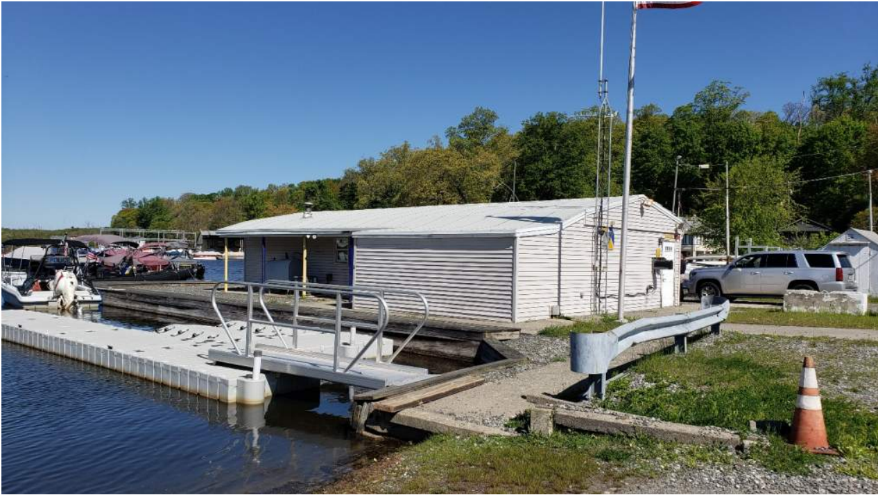
Existing Police Station Building – South and East Facades
