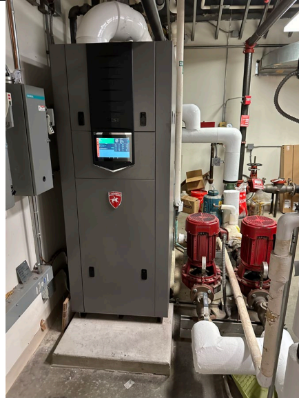
Existing Lockinvar boiler and pumps
