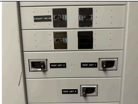
Existing panel PP3 on third floor with RTU and toilet EF breakers.
