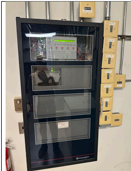
Existing Notifier fire alarm control panel
