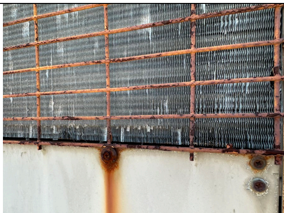
Typical coil degradation
