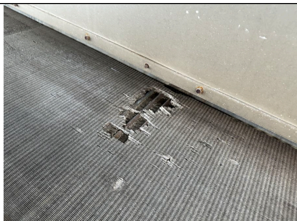
Typical coil degradation
