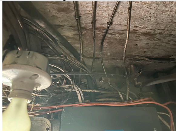
Typical wiring and cut-off hot water pipes
