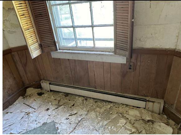
Typical fin tube radiation
