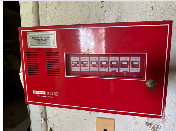
Fire alarm control panel
