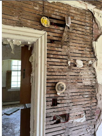
Typical fire alarm devices on the wall
