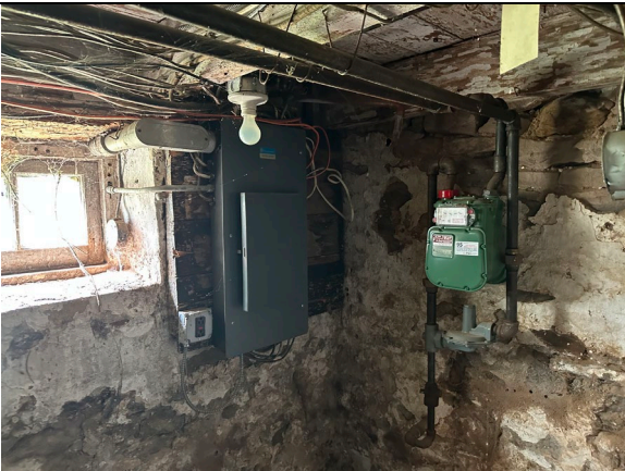
Gas meter and electrical panel
