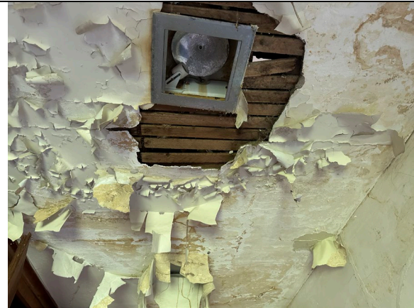
Recessed ceiling incandescent fixture
