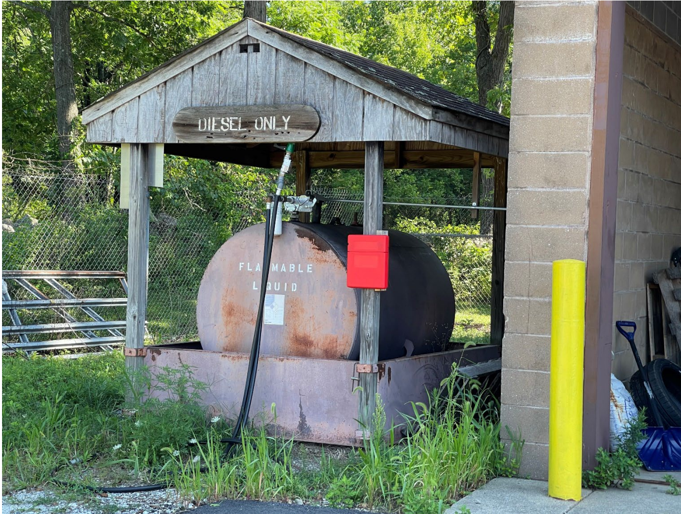
The existing 500 gallon diesel fuel above ground storage tank.
