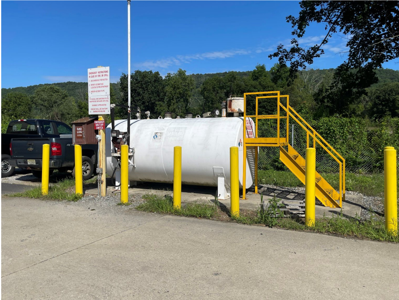
The Existing 2000 gallon gasoline above ground storage tank.
