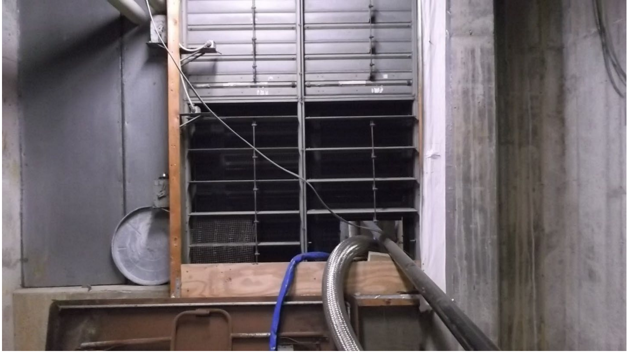
Basement louver to be temporarily removed to facilitate boiler removal and replacement.
