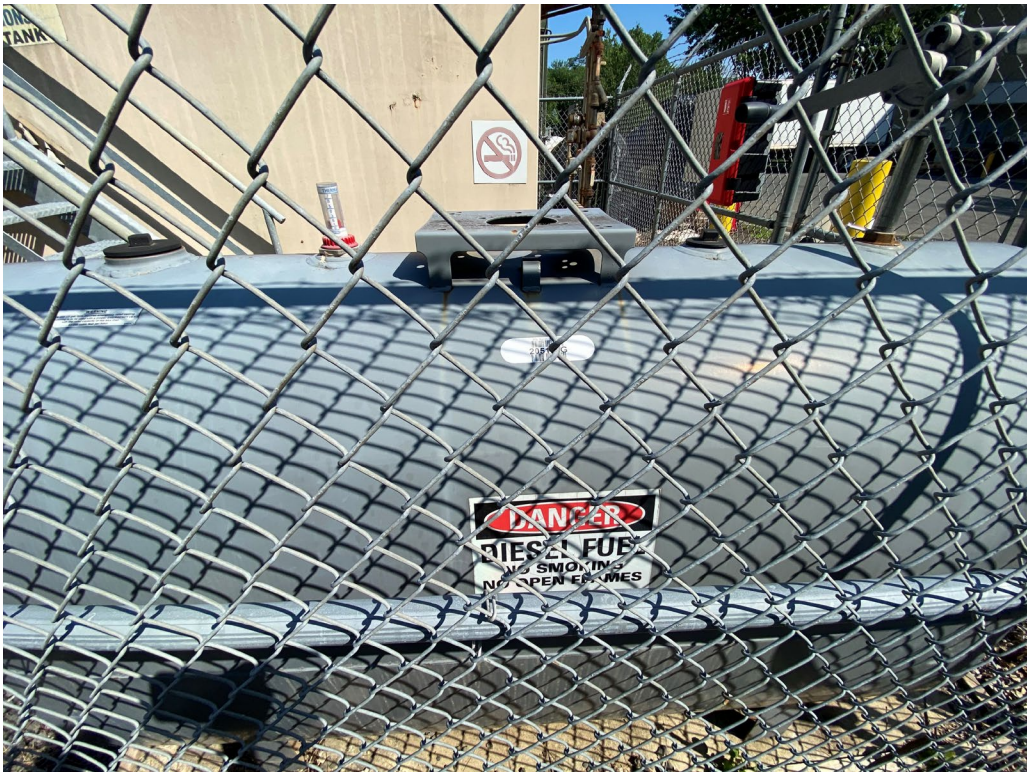
Photo 15 – 330-Gallon Diesel AST
