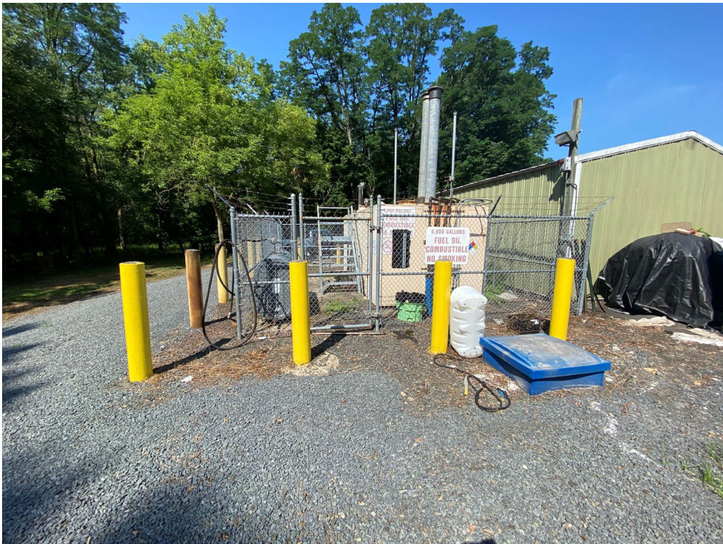
Photo 17 – AST Containment Traffic Protection
