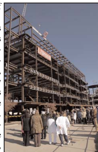
Meridian expansion construction site
