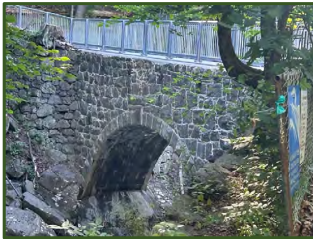
Figure 20: The Arch Bridge 5
