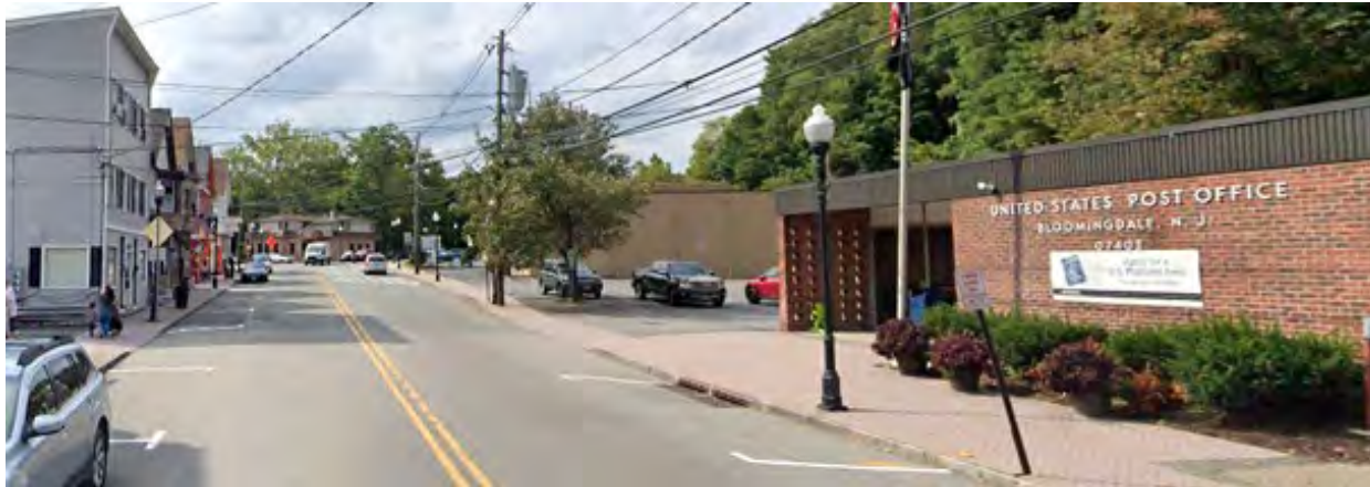
Figure 13: Consumers may feel unsafe by narrow sidewalks and close proximity to vehicle traffic.
