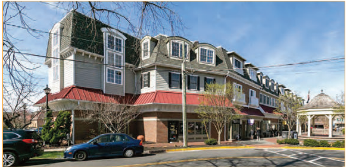
Upscale condominiums above retail shops at Kings Court in downtown Haddonfield, New Jersey.
