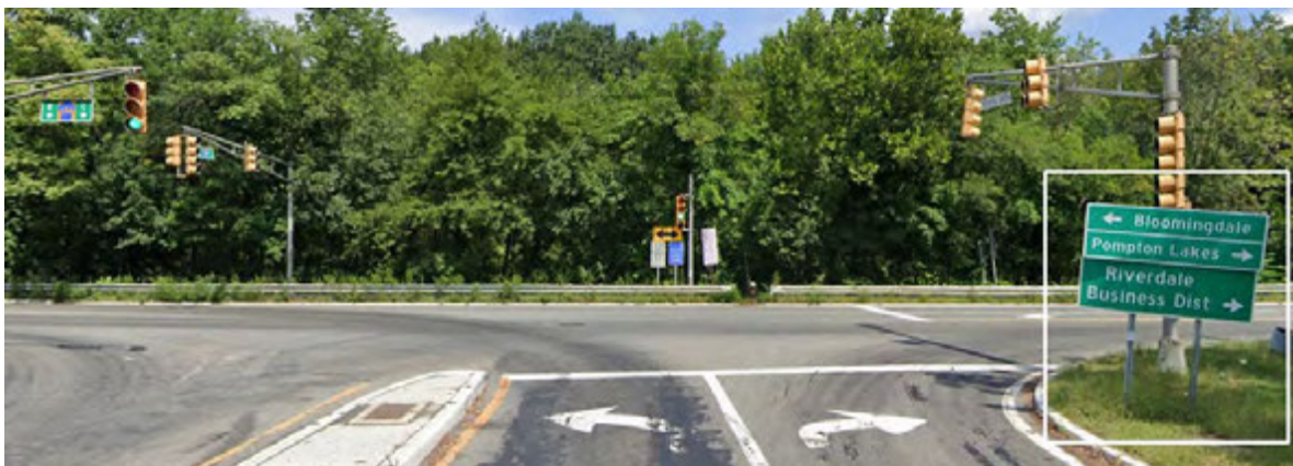
Figure 8: South-bound off-ramp of I-287 looking toward Hamburg Turnpike.
