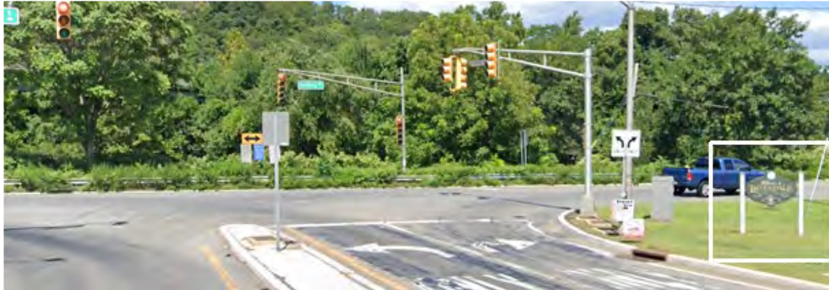
Figure 9: Off-ramp of I-287 north-bound facing Hamburg Turnpike.
