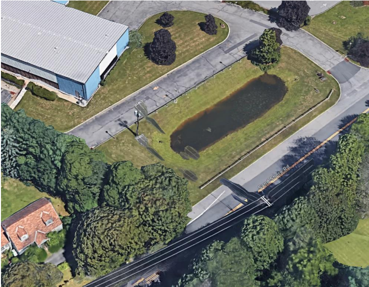
Block 8300, Lot 9 Retention Pond
