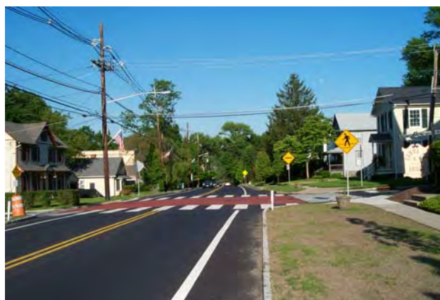
Traffic calming improvements in Rocky Hill
