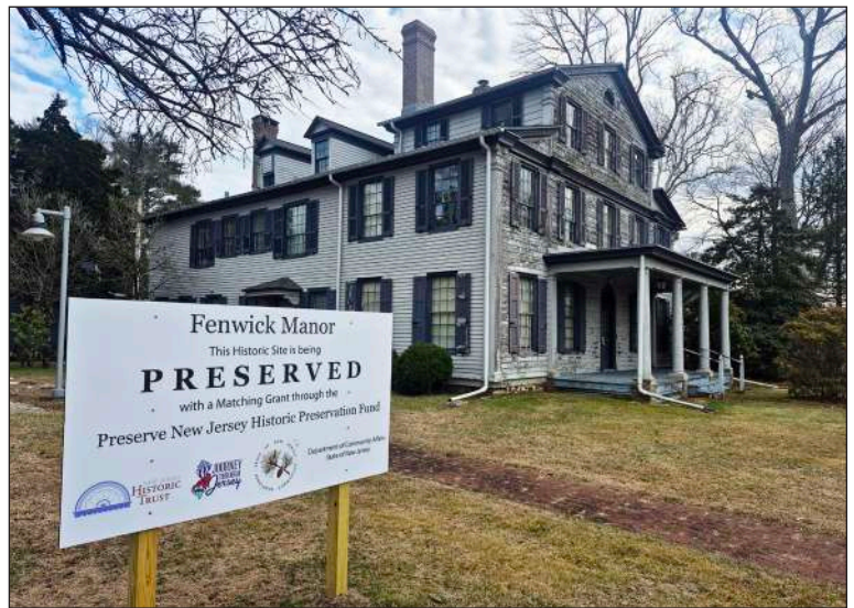
Above: In 2025, the Commission took significant strides toward rehabilitating one of its principal office buildings, Fenwick Manor.
