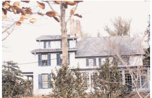
Fenwick Manor is located amidst a serene setting along Springfield Road in Pemberton Township.
