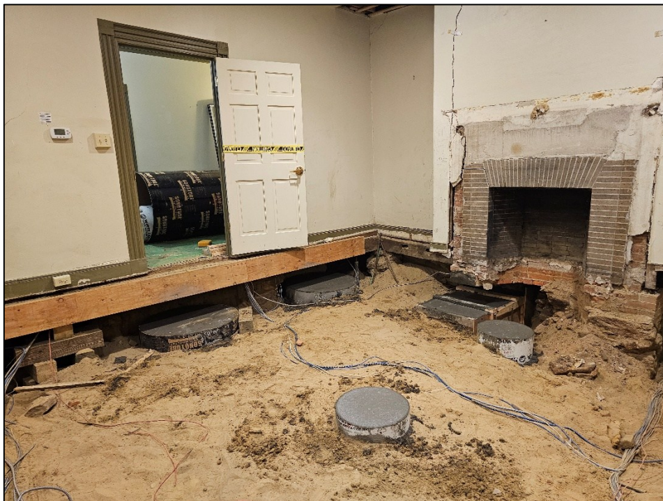
Above: New concrete foundation piers in the Executive Director's office.
