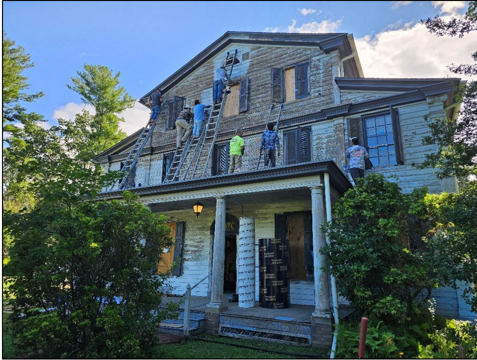
Above: Exterior surface preparation underway on Fenwick Manor's street facing elevation.
