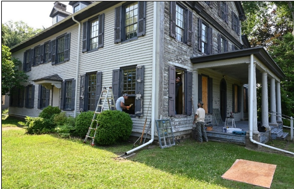
Above: Contractors with Hawley Bros. started to remove the historic windows from the Fenwick Manor farmhouse on June 30, 2026. The windows will be restored and reinstalled as part of the project.
