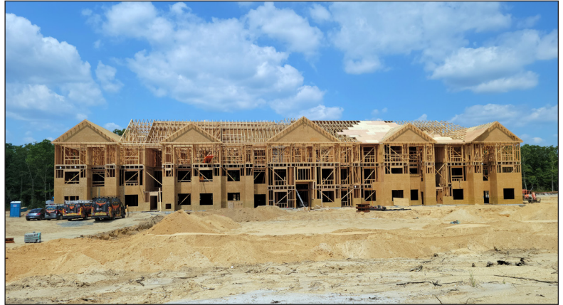
Above: This 148-unit, age-restricted condo development is being built in Barnegat Township, Ocean County, with the use of 7.5 Pinelands Development Credits. The development will also include a 2,688-square-foot clubhouse. Photo/Paul Leakan
