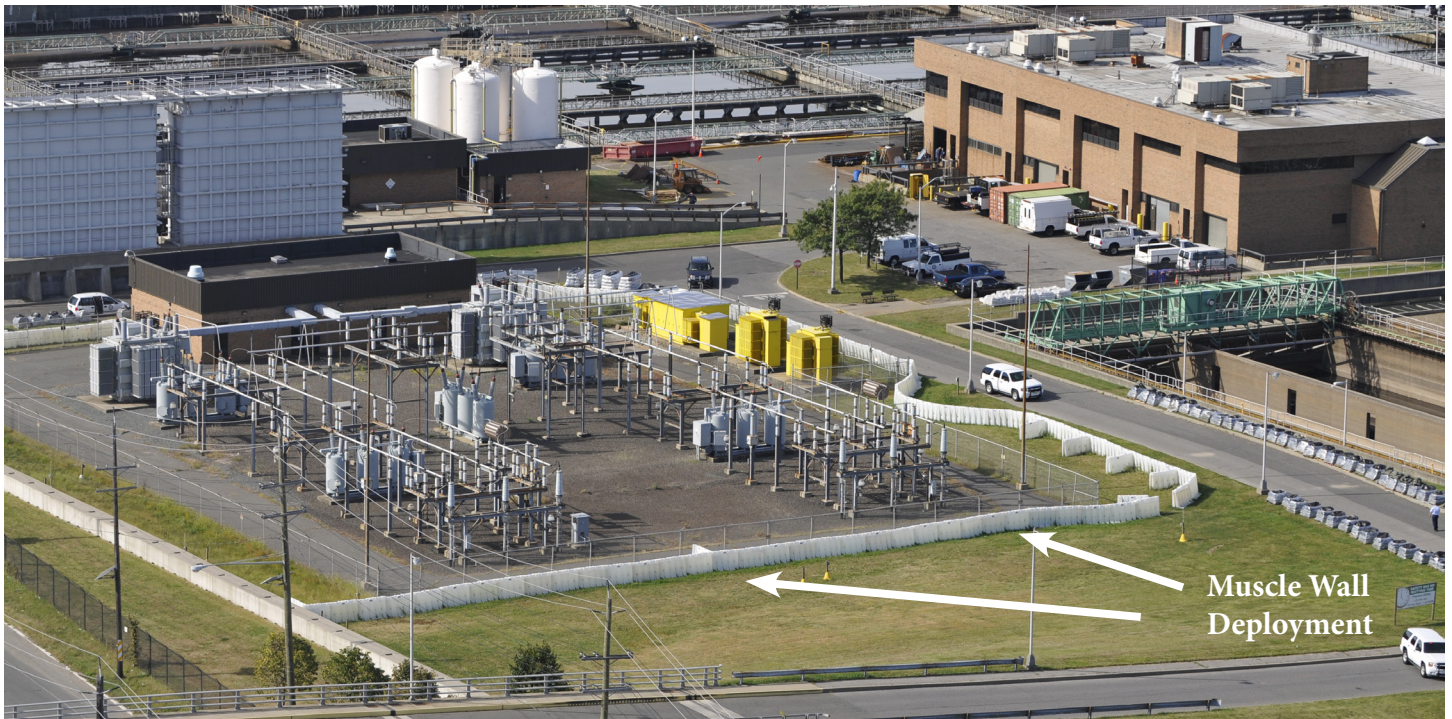
Muscle Wall flood barrier deployed around PVSC electrical substation
