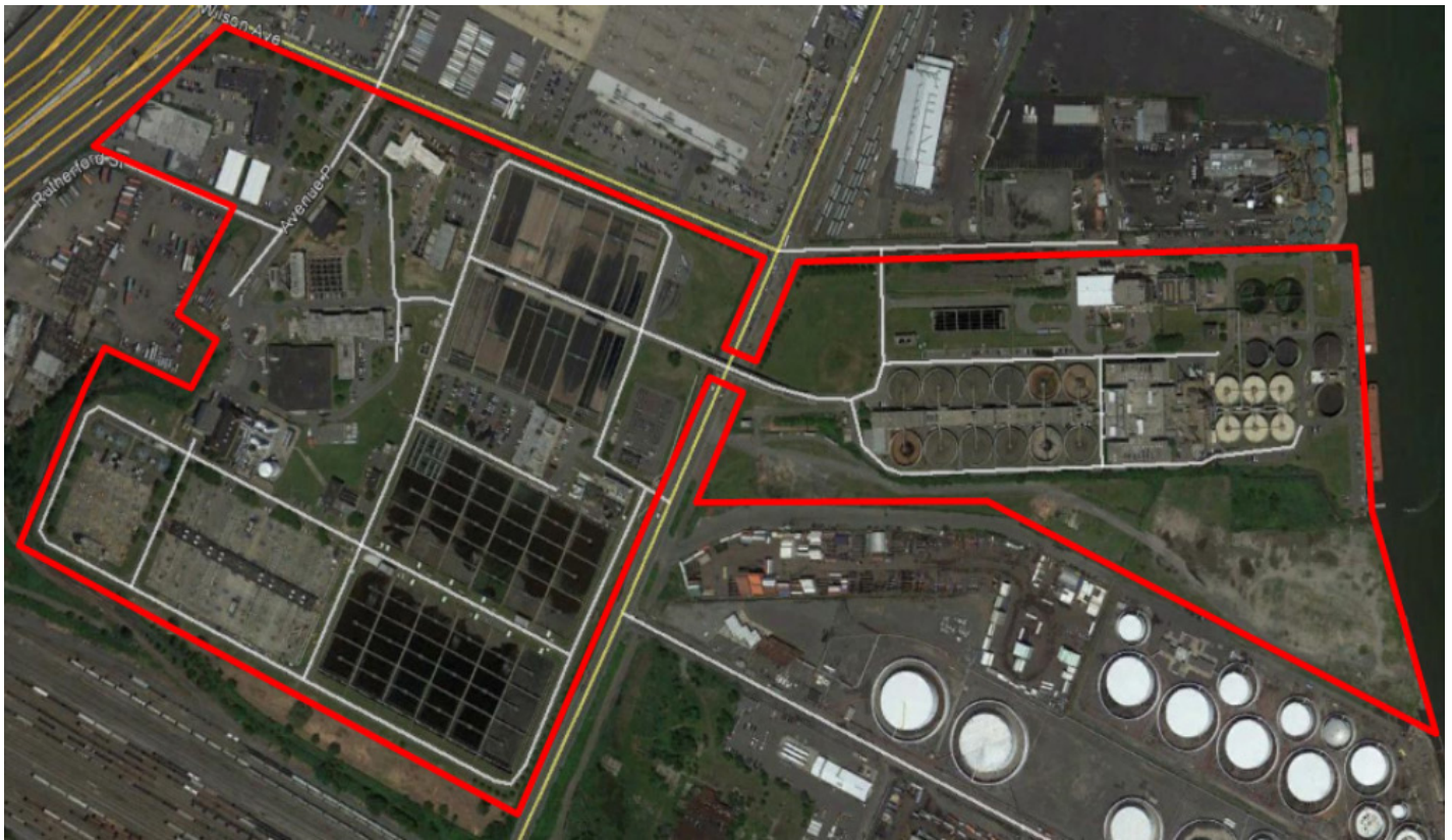
Aerial view of the Passaic Valley Sewerage Commission
