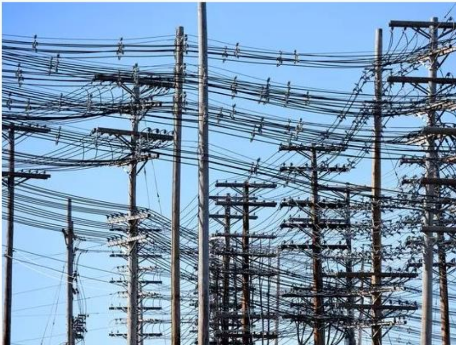
Since the Passaic Valley Sewerage Commission plant lost electricity during Superstorm Sandy they have moved all of their electricity from underground to above ground at their Newark plant. (Photo: Amy Newman/NorthJersey.com)
