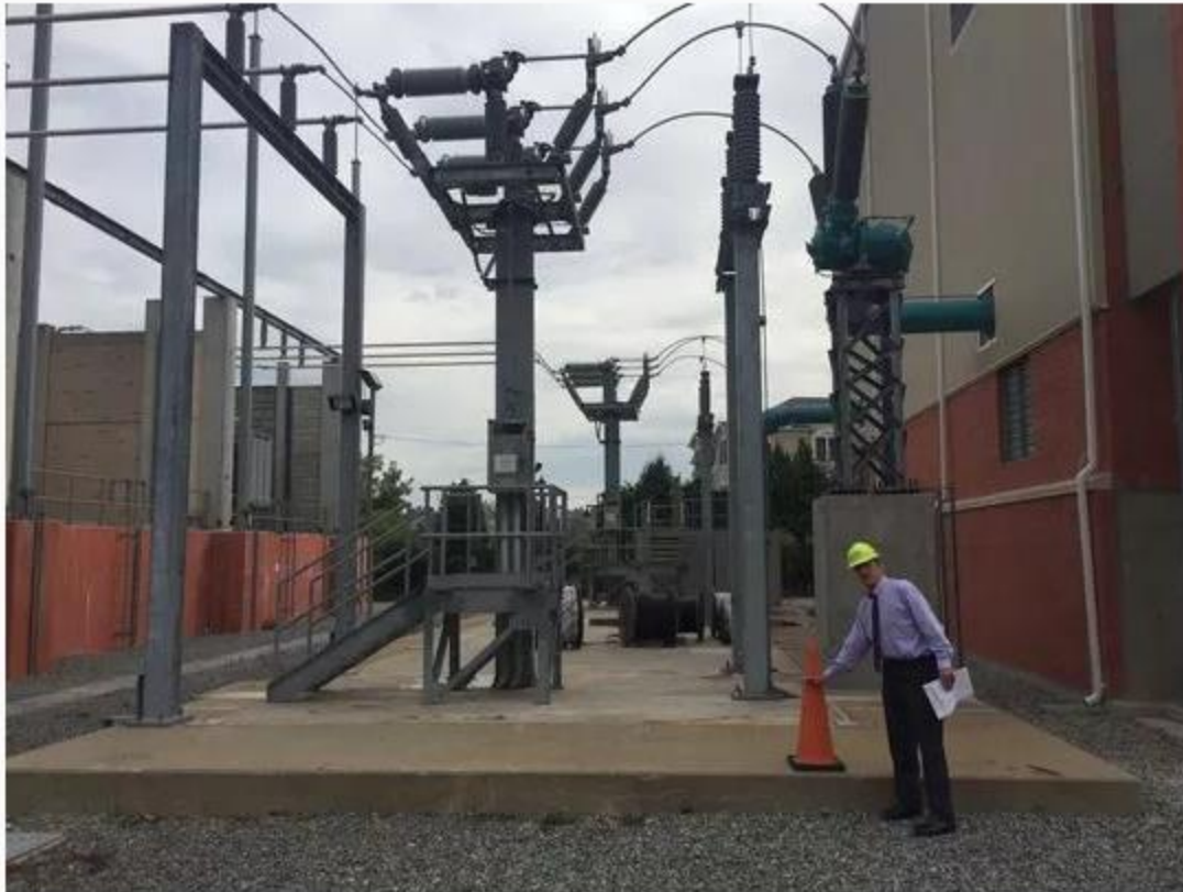
PSE&G's John Latka shows how high the storm surge from Sandy got at the substation in North Bergen along the Hudson River. Key equipment that had rested on the concrete pad has since been elevated far above that level to make the system more resilient in future storms. (Photo: James M. O'Neill/NorthJersey.com)
