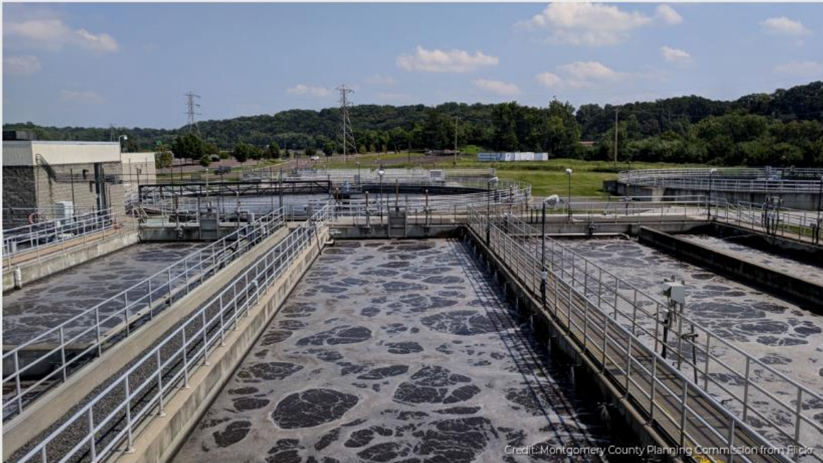
An aeration tank at a wastewater treatment facility
