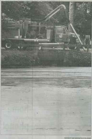
Workers from the Passaic Valley Sewerage Commission, including Alex Hernandez, below left, and George Krusznis use a vacuum truck, above, to clean out a dam in the north pond of Branch Brook Park. The blockage of the dam and drainage system has prevented water in the pond from going in and out of the main lake and the water has become stagnant and covered with algae and duckweed. Essex County parks workers also have begun skimming the surface of the pond to clean it.
