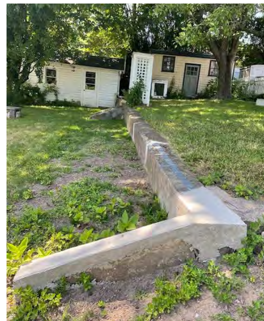
TOP: Restored cold frames at Botto House. ABOVE: The historic site of the cold frames prior to reconstruction.
