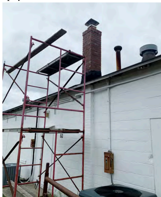
TOP: Millville Army Airfield Museum. ABOVE: Scaffolding stands at Base Headquarters amid work on the museum’s chimneys in summer 2024.
