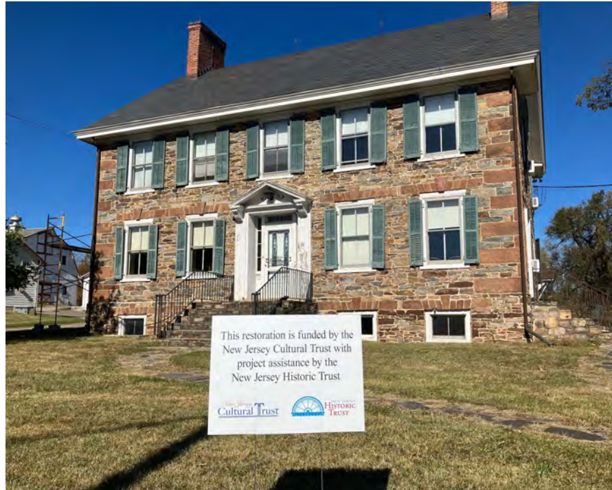
ABOVE: Case-Dvoor Farmstead, Hunterdon Land Trust (Hunterdon County). Hunterdon Land Trust was awarded a $40,000 CHP grant in FY24 for repointing and plaster repair.
