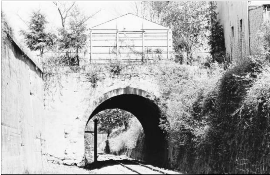
Railroad Underpass, Farnsworth Avenue, Bordentown, Burlington County
